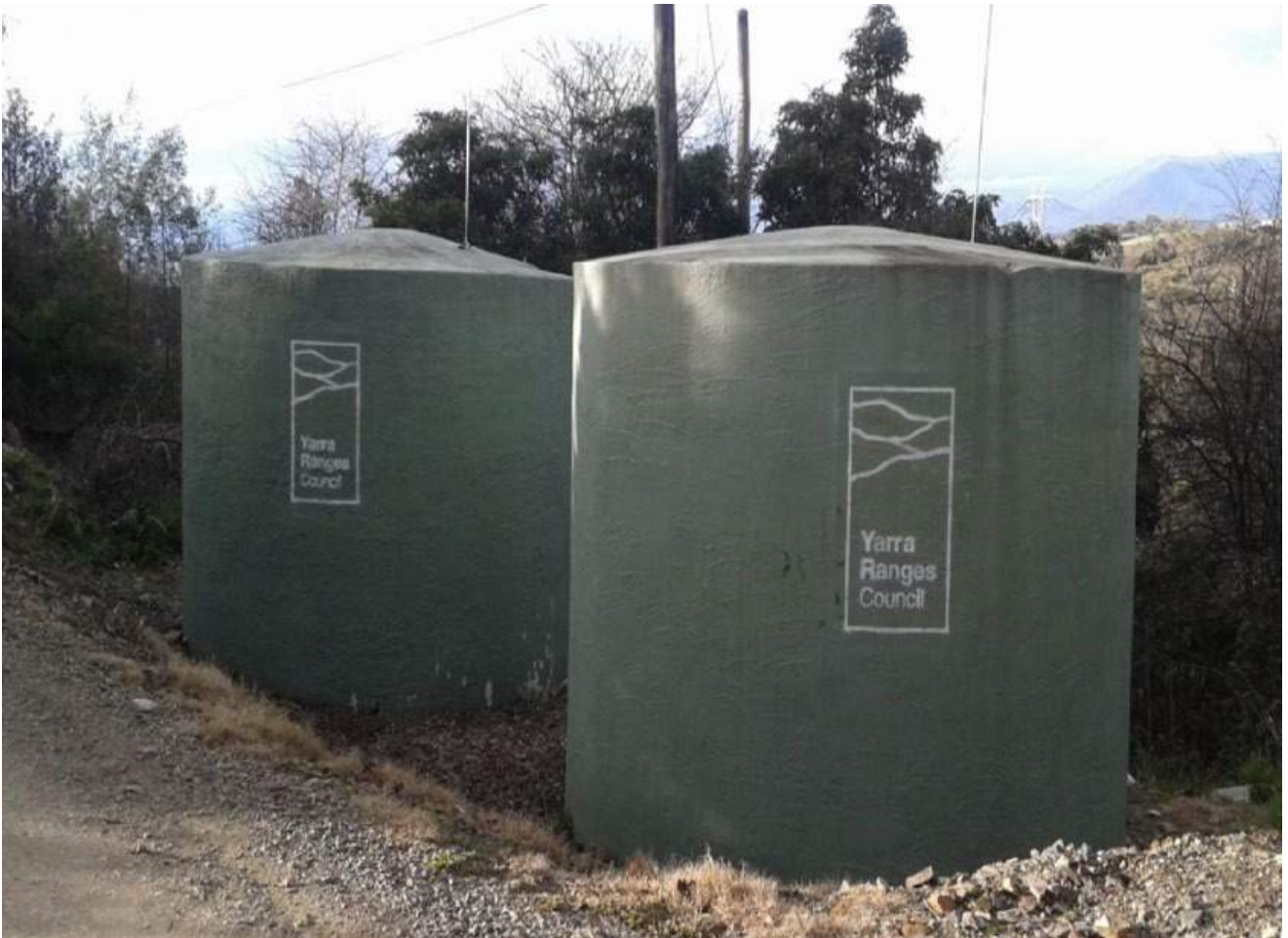
Figure 29 - Roadside static water supplies for firefighting purposes in the Yarra Ranges, Victoria (Source: Yarra Ranges Council, 2013)
