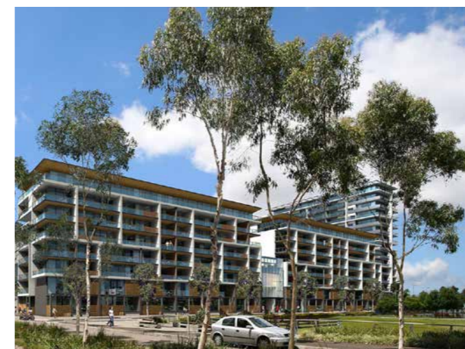
Figure 25: Proposed location of high rise residential, and desired character and built form
