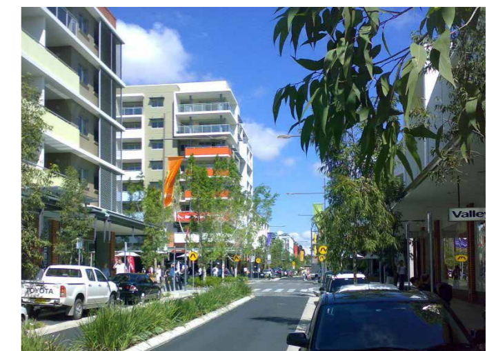
Figure 26: Proposed location of mixed use retail & residential, and desired character and built form
