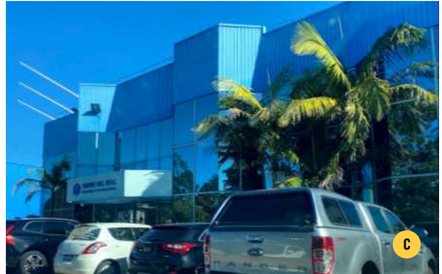
An example of older, yet well-maintained, strata office/warehouse units within the Precinct (Map 2.4C).
