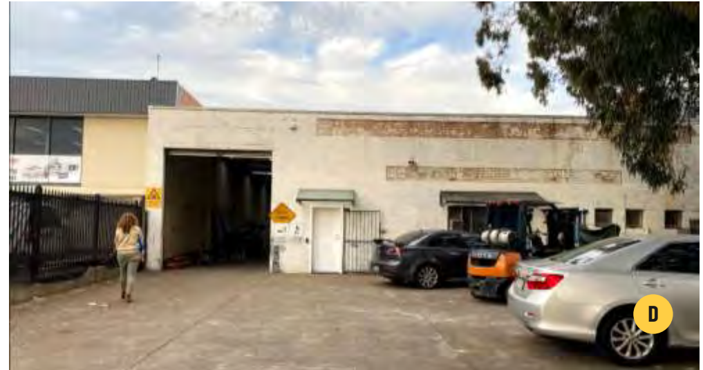
Older warehouses typically seen within the Precinct.
