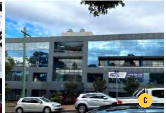
Most buildings in the Precinct contain office uses fronting the main street and warehousing to the rear (Map 1.4C).
