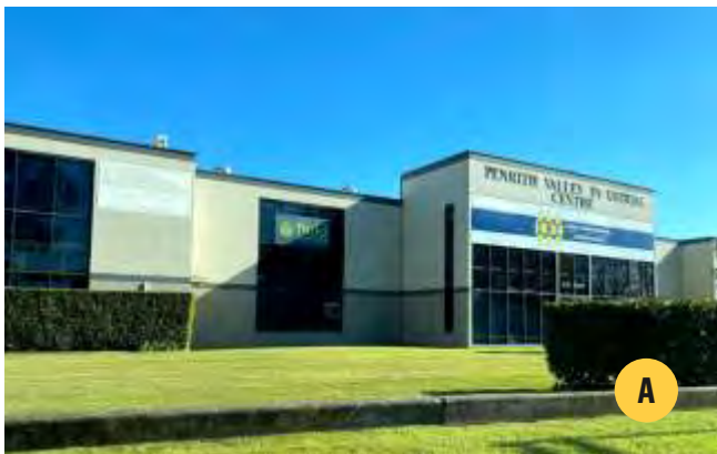
Older style strata warehouses with ancillary office uses found along Borec Road (Map 1.4A).
