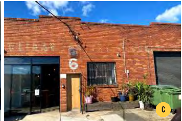
An industrial warehouse conversion for use as a gin distillery and bar (Map 3.C).
