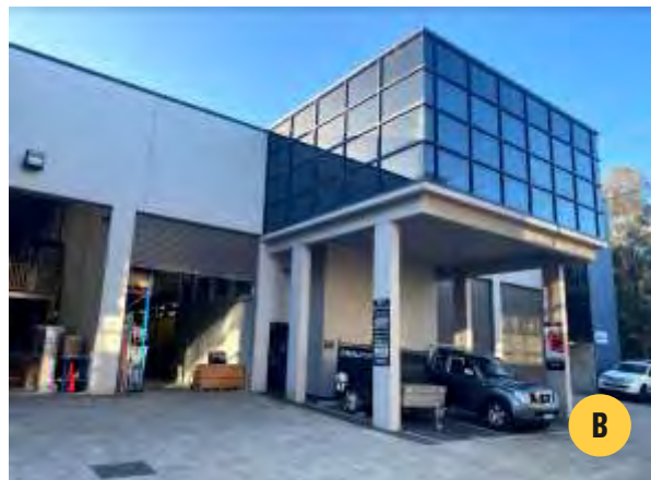
The Precinct features some modern developments, including this strata office/warehouse (Map 1.4C).
