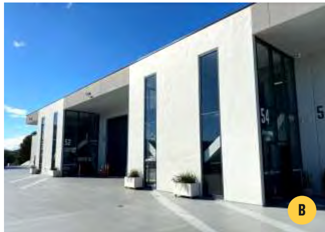
New strata warehouse unit complex at 76B Edinburgh Road (Map 3.B).
