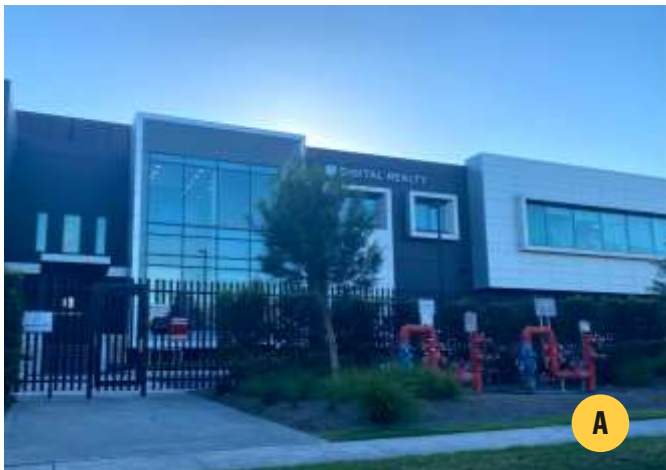
One of Digital Realty's existing data centres located along Templar Road (Map 1.4B).
