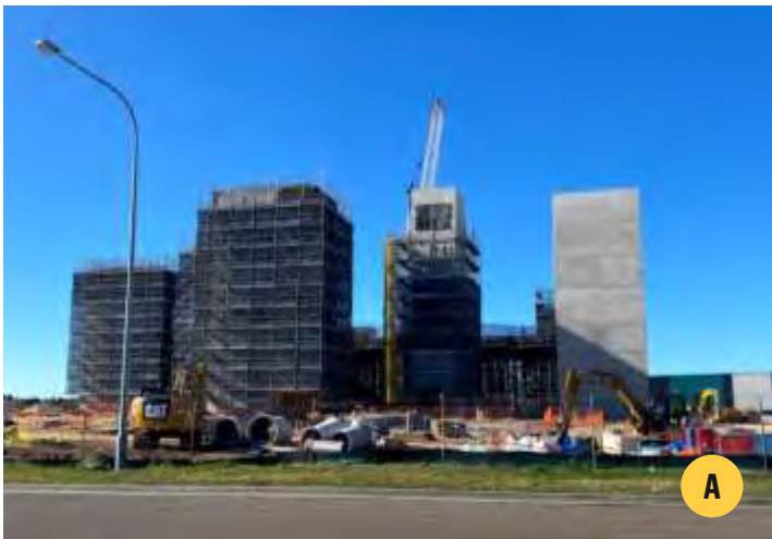
Data centre currently under construction at 10 Eastern Creek Drive (Map 1.4A).
