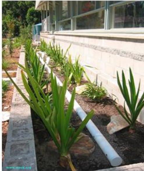
Planter box bio-retention system, Sydney
