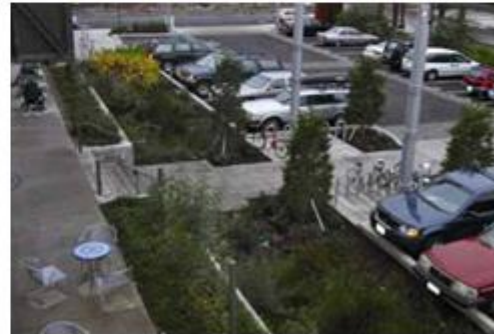
Planter boxes can treat stormwater from paved areas, USA
