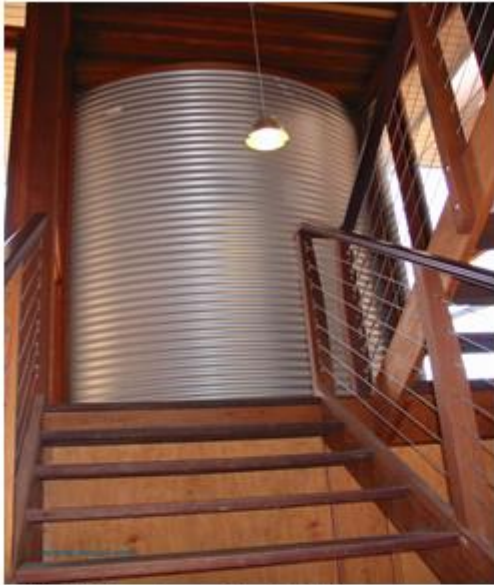
Initial planning of the building footprint should allow adequate space for rainwater tanks.
