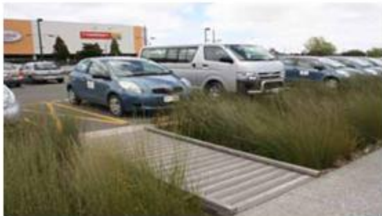
Raingardens in car-park, New Zealand
