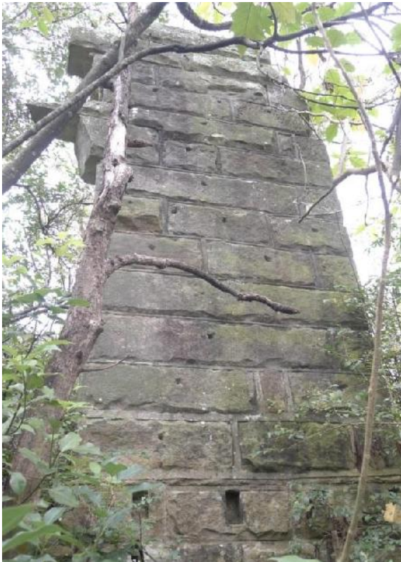
Figure 3.11 Detailed view of the sandstone wall relating to the Powderworks, believed to be part of the original Office and Magazine building. Checkouts are visible for possible timber joists and indentions indicate the position of a structure that was previously fixed to the wall. (Source: GML 2014)
