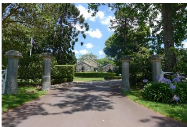
Figure 3.2 View of Ingleside House from Manor Road, showing the sandstone entry pillars, carriage loop and east elevation of the house. (Source: GML 2014)
