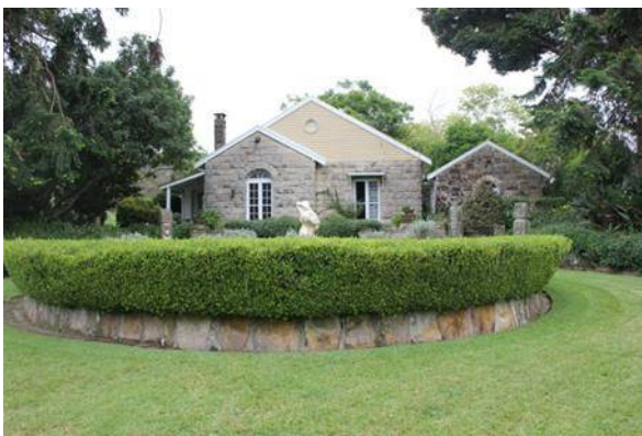
Figure 3.4 East elevation of Ingleside House. The carriage loop is no longer used to convey vehicles. The additional sandstone wing is visible on the right. (Source: GML 2014)
