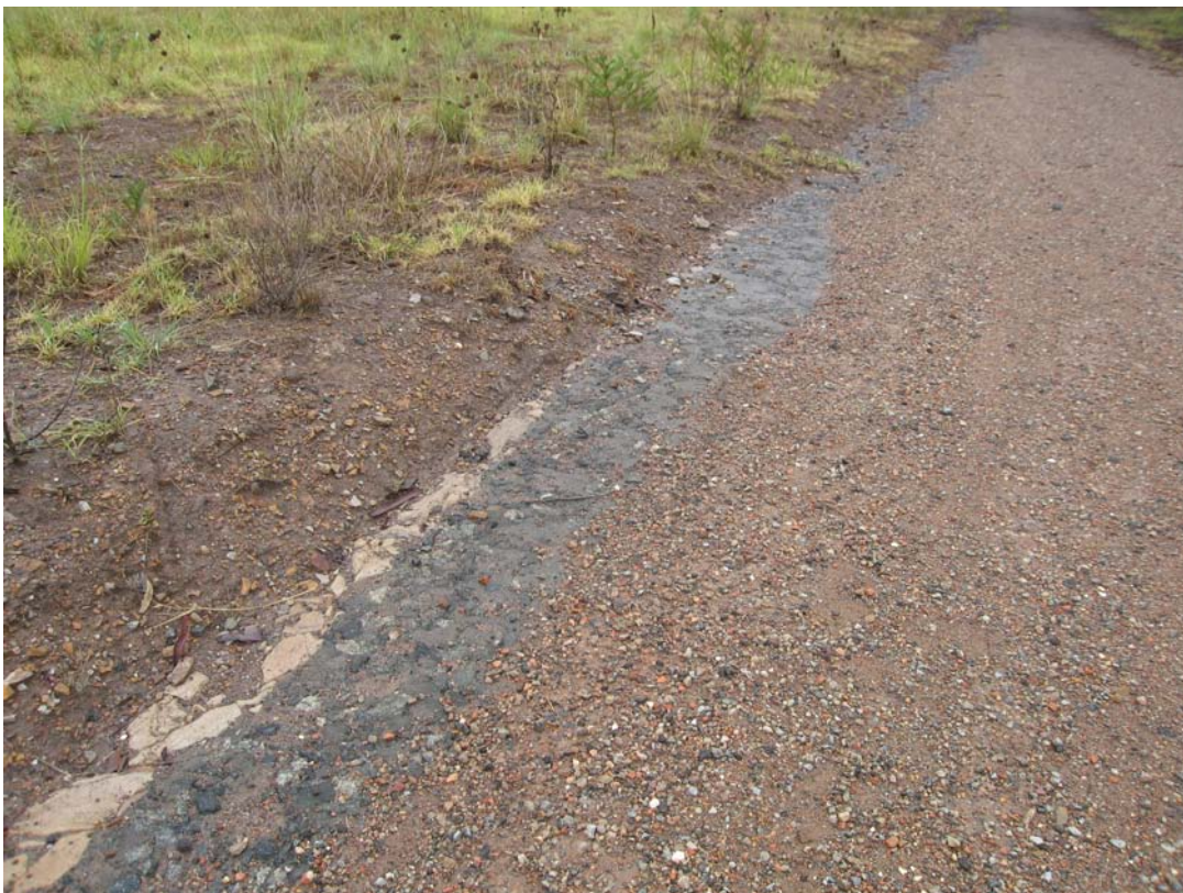
Figure 5.2 Sandstone remnants of earlier Windsor Road surface, looking south. (Source: GML 2009)
