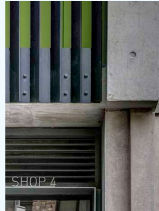
Designed to last Face brick, off-form concrete and steel detailing provide robust, low-maintenance and long-life quality. Images Brett Boardman Photography.
