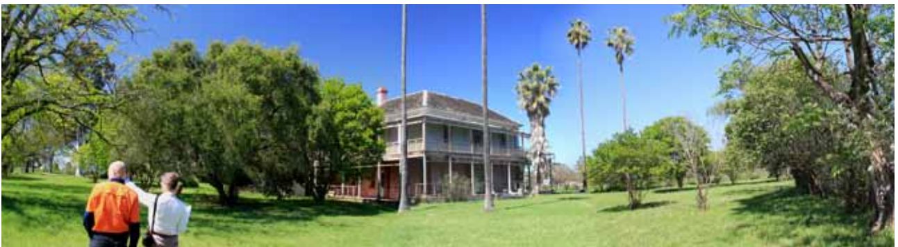
Plate 11 View looking south to Clydesdale House from within the House garden
