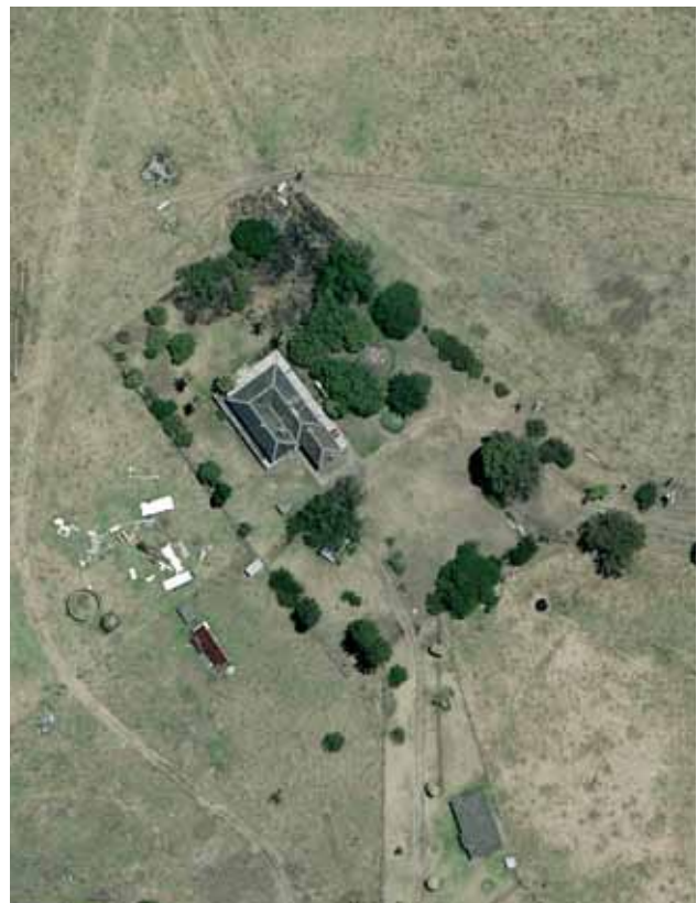
Plate 30 Aerial photo of Clydesdale House and garden. Note the multiple exotic trees planted in close proximity to the house, which limits views to the surrounding landscape
