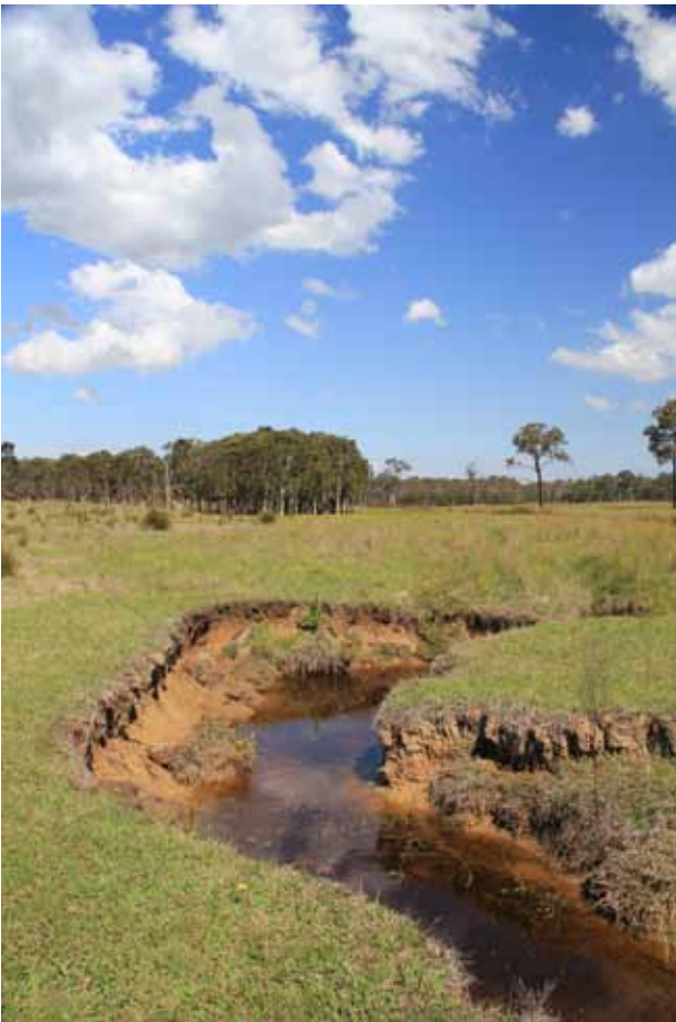
Plate 1 Erosion in a watercourse on site
