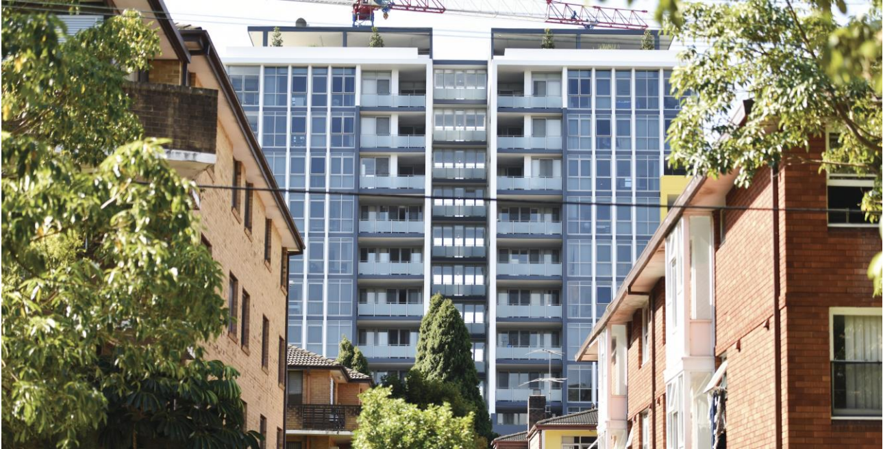
Figure 3. Apartment construction in Strathfield in Sydney's Inner West
