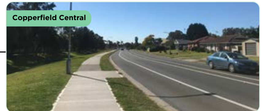
Figure 4: Looking north up Copperfield Drive.
