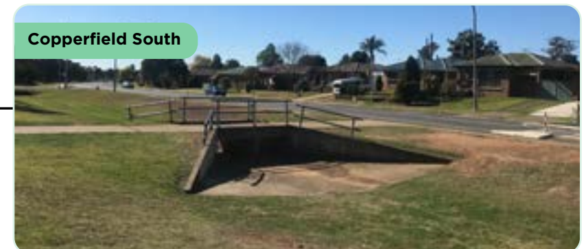
Figure 5: Drainage channel crossing from Copperfield Drive to Rosemeadow Public School.
