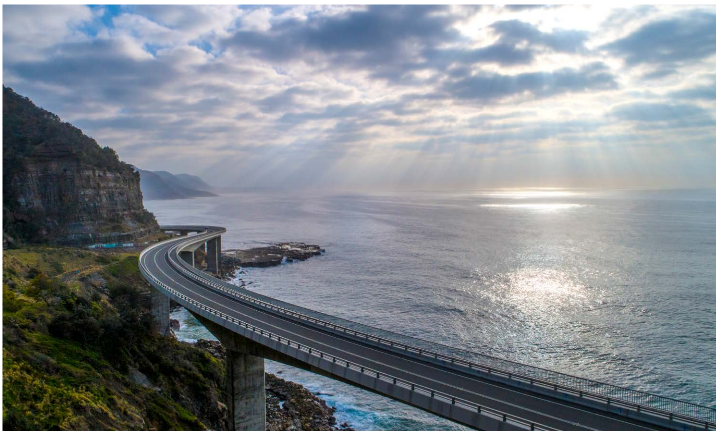
Sea Cliff Bridge, Clifton –City of Wollongong LGA / Tharawal Country (Photography: Destination NSW)
