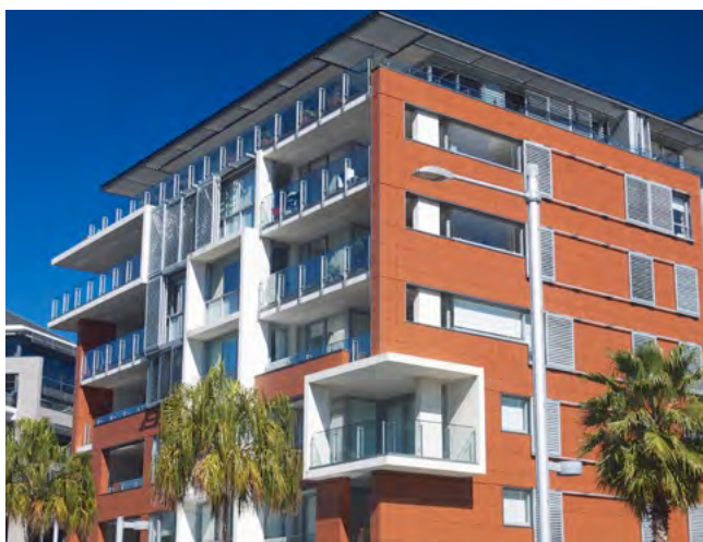
Figure 4M.4 The terracotta tile cladding used on this building contrasts with the white framed balconies and roof line, adding visual interest
