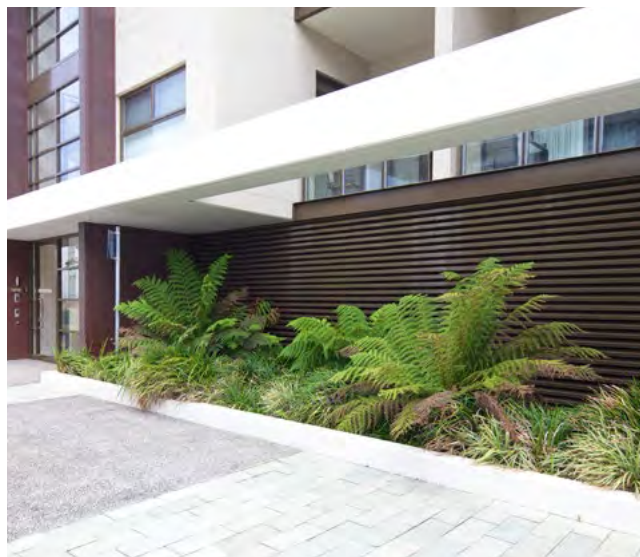
Figure 4W.2 Common waste and recycling areas should be screened from view and well ventilated
