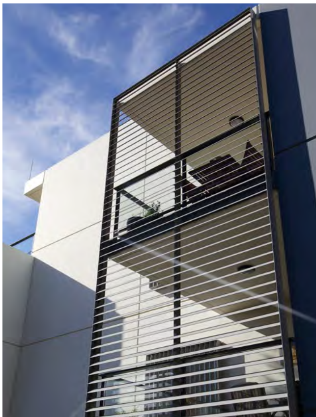
Figure 4A.3 Horizontal louvres are most effective on north facing elevations and achieve summer shade and winter sun access
