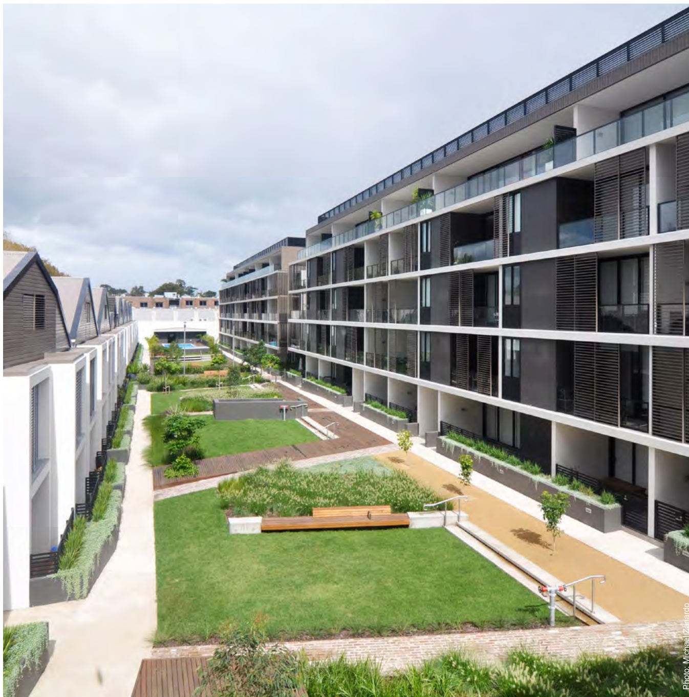
Figure 3D.11 Attractive and inviting communal open spaces with good solar access should be provided
