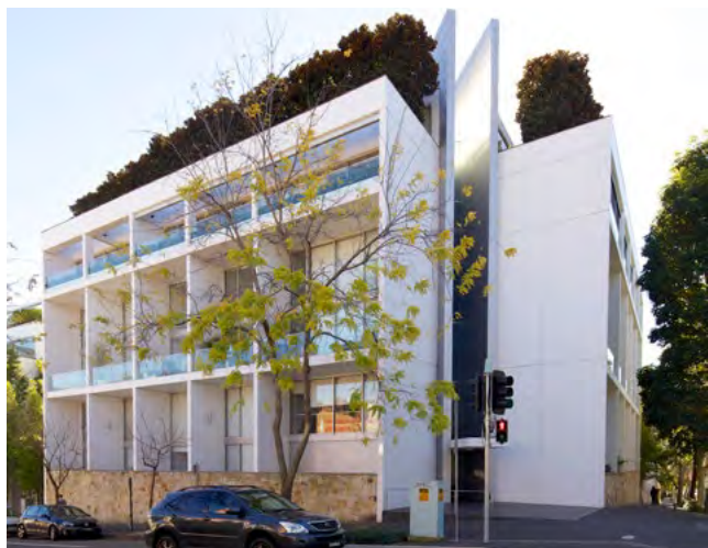
Figure 4M.5 Changing facade materials, building articulation or height effectively highlights prominent corners
