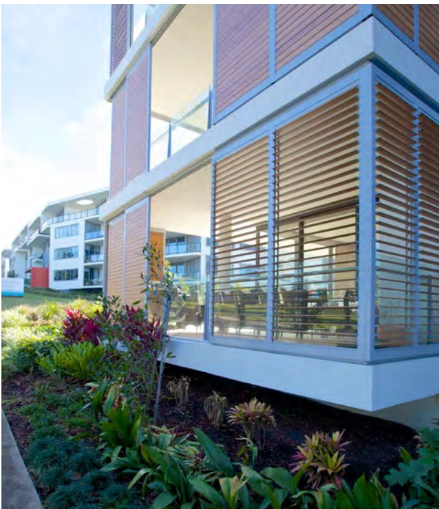
Figure 4E.5 Primary balconies provide outdoor living, articulate the building facade and contribute to the safety of the public domain through increased surveillance opportunities
