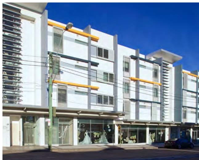
Figure 4J.1 Where balconies are oriented away from a noise source, changes in facade texture and detail along the busy road can assist in dispersing noise. This mixed use development is located on a busy road and is designed with limited openings exposed to the noise source
