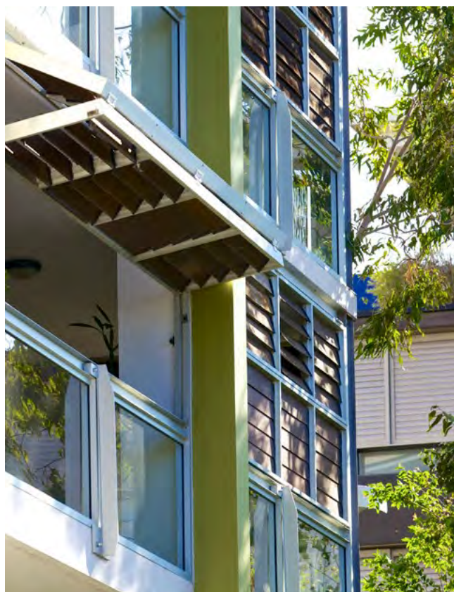
Figure 4A.8 Trees help shade building facades. For east and west facing facades consider planting deciduous species
