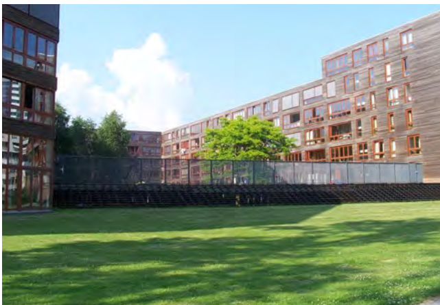
Figure 3J.6 Natural ventilation to the underground car park is integrated into the landscape design of this development
