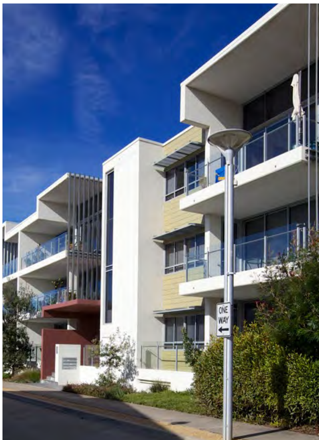
Figure 4X.3 Roof overhangs, hoods and drip lines protect walls from the elements (rain, sun and wind) reducing maintenance costs
