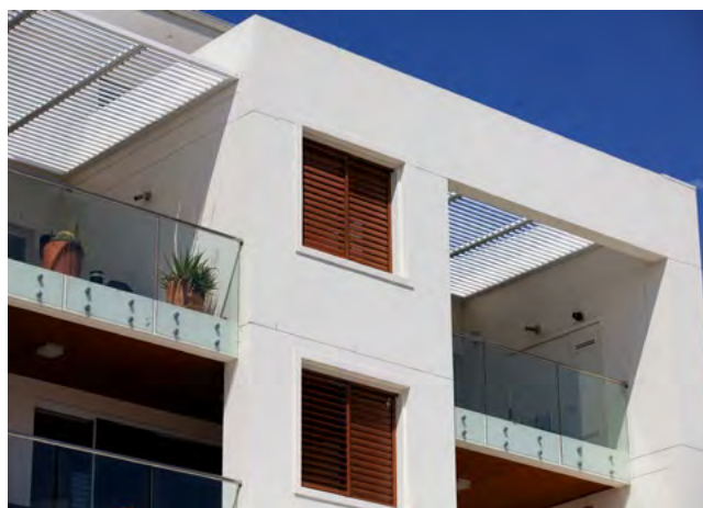
Figure 4H.1 Appropriate finishes, treatments and construction methods help reduce noise transmission through walls and floors
