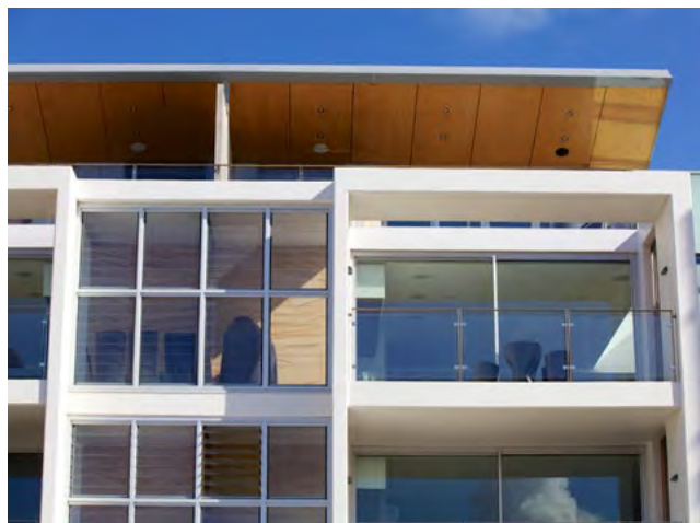
Figure 4N.2 Architectural roof features and articulation are generally allowed to exceed the maximum statutory building height
