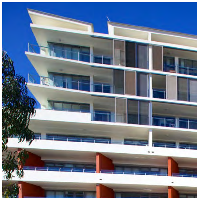
Figure 4A.5 At least 70% of all apartments in a building should receive a minimum of 2 hours direct sunlight in mid winter in the Sydney Metropolitan Area and in the Newcastle and Wollongong local government areas, and at least 3 hours direct sunlight elsewhere in NSW
