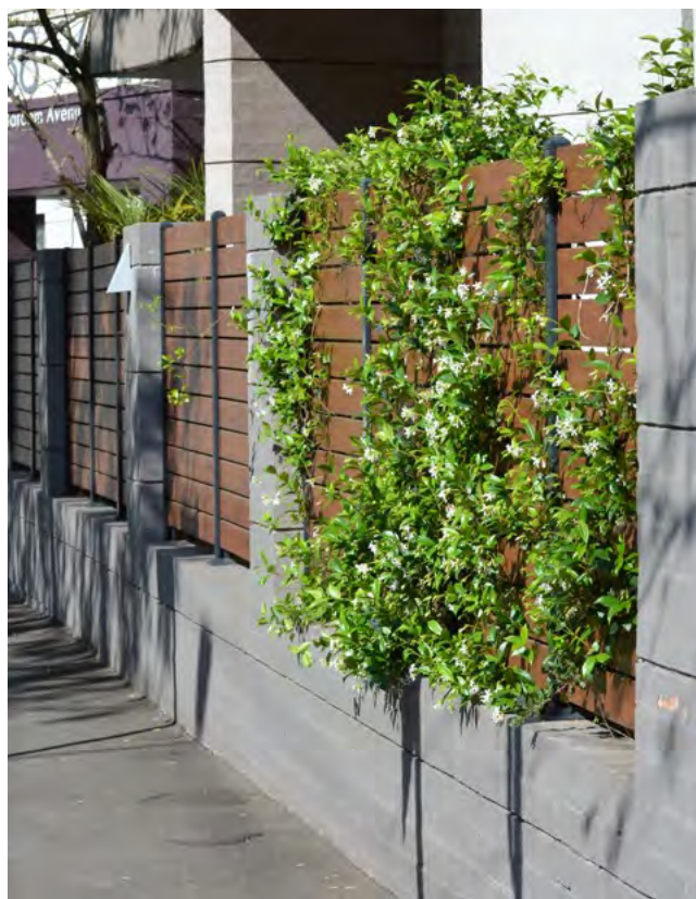
Figure 3C.4 Front fences along public street frontages should use visually permeable materials and treatments such as timber slats
