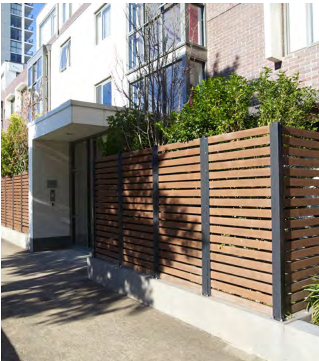
Figure 4G.3 Storage located on private balconies or within courtyards should be fully integrated and screened from view
