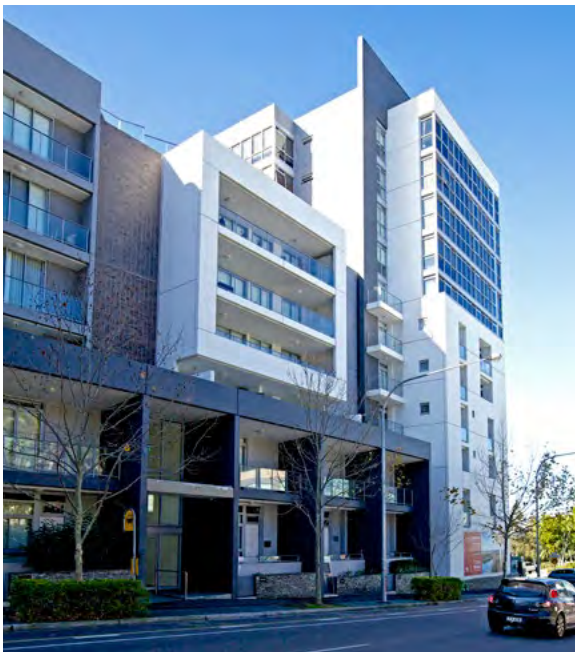
Figure 2E.3 Building depth dimensions should include articulation such as projecting balconies, gallery access, overhangs, blades and other architectural features
