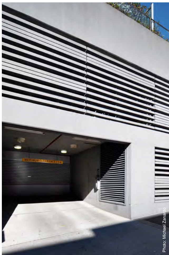
Figure 3J.16 Screening can be used to integrate above ground car parking with the facade
