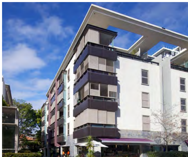
Figure 4N.1 Special roof features need to be proportionate to the overall building size, scale and form
