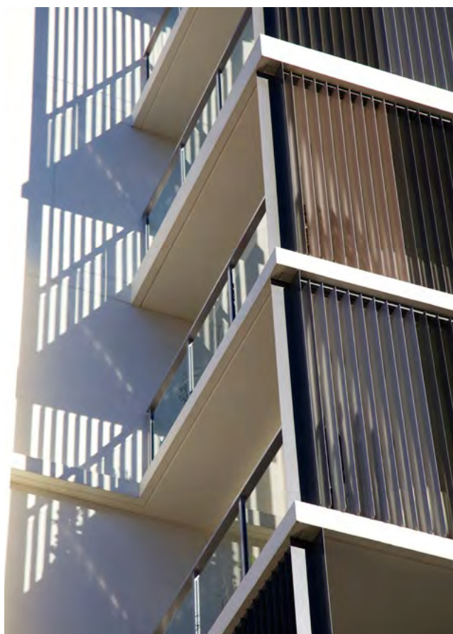
Figure 4A.7 Vertical louvres are an effective sun management technique for east and west-facing windows and balconies
