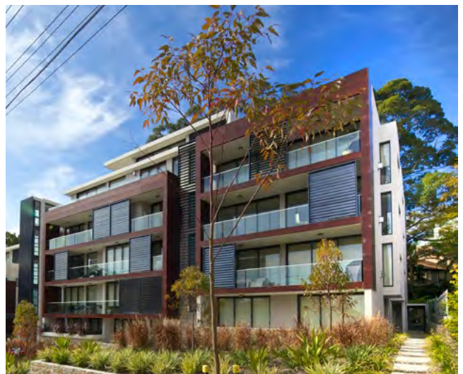
Figure 2H.1 Side setbacks can contribute to the character of the street, for example by allowing views to existing vegetation at the rear of buildings
