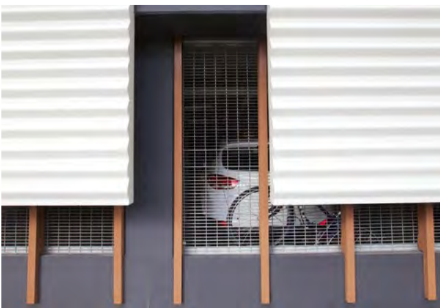
Figure 3J.12 Where car parks are located above ground and visible from public or common areas, they should be partially or fully screened from view
