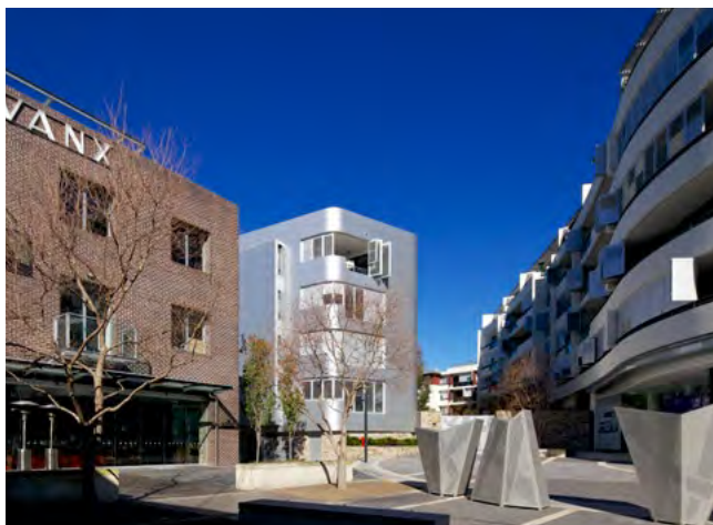
Figure 4R.4 Contemporary infill can create an interesting dialogue between old and new, adding to the character of a place
