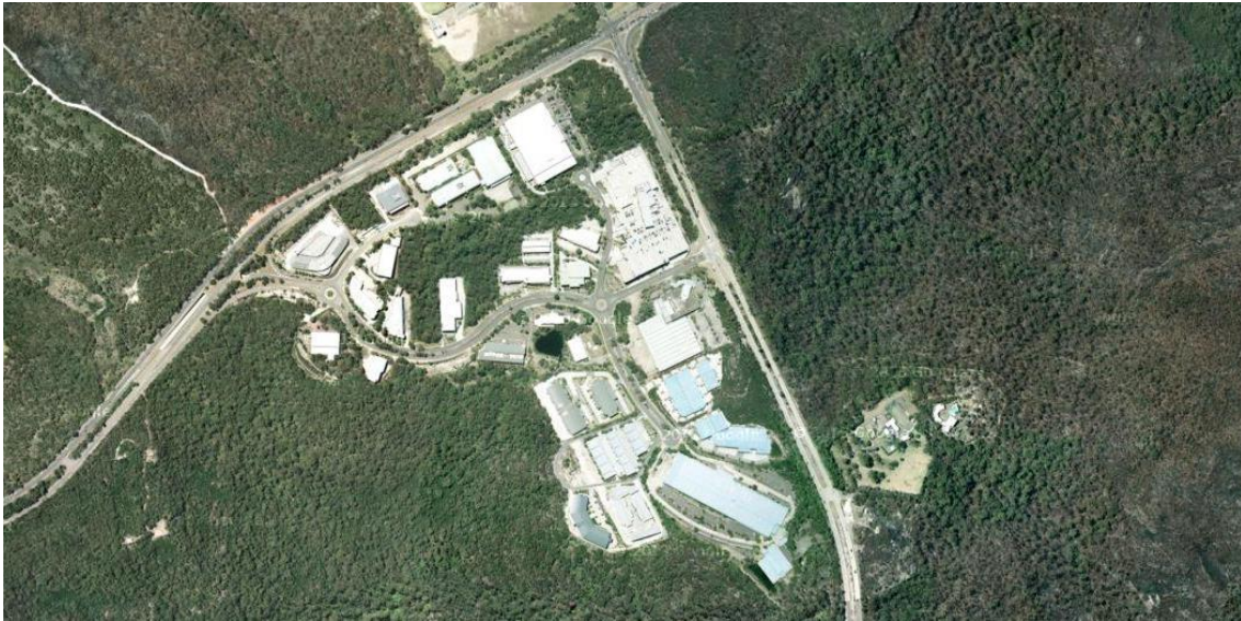
FIGURE 10. AERIAL OF BELROSE (AUSTLINK BUSINESS PARK)
