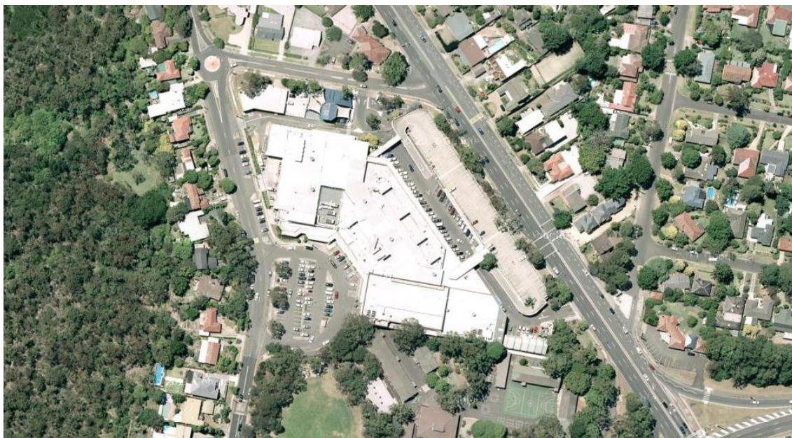
FIGURE 24. AERIAL OF FOREST WAY
