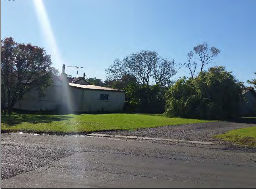
POTENTIAL HAZARDOUS MATERIALS IN SHEDS ALONG ARNOLD AVENUE
