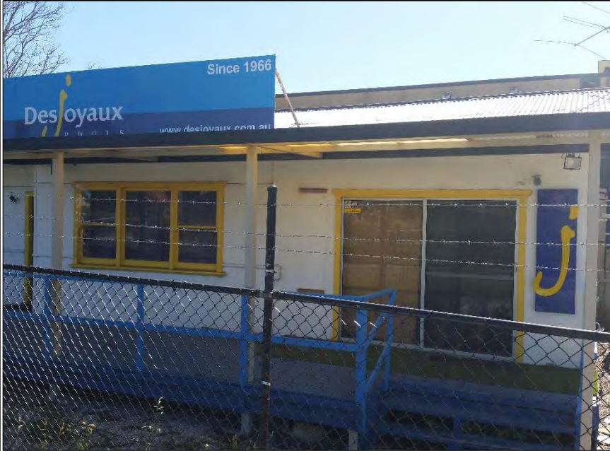
POTENTIAL HAZARDOUS MATERIALS BUILDING AT THE LANDSCAPE SUPPLIERS YARD
