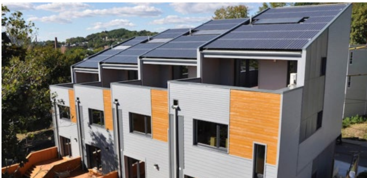
Figure 3-124 Roof mounted photovoltaics should be integrated into the design of the dwelling
