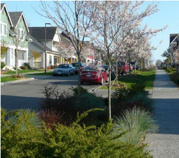
Figure 3-129 Swales can be attractive, and are able to filter and collect the stormwater
