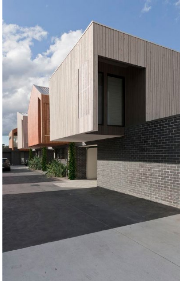
Figure 3-100 A poor acoustic outcome is achieved when driveways are in close proximity to bedrooms and living rooms, and driveways are hard paved reverberating sound.
