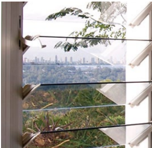
Figure 3-69 Operable louvres allow residents to regulate natural ventilation
