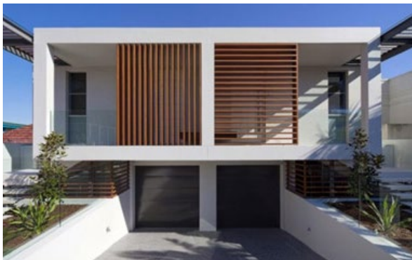
Figure 3-99 Privacy screens can be an integral part of the articulation. Changing the pattern and direction of the screen adds visual interest and asymmetry to the facade.
