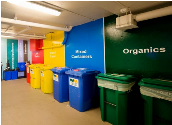
Figure 3-136 Well designed, easily accessible and clean waste and recycling rooms improve the collection and management of household waste
