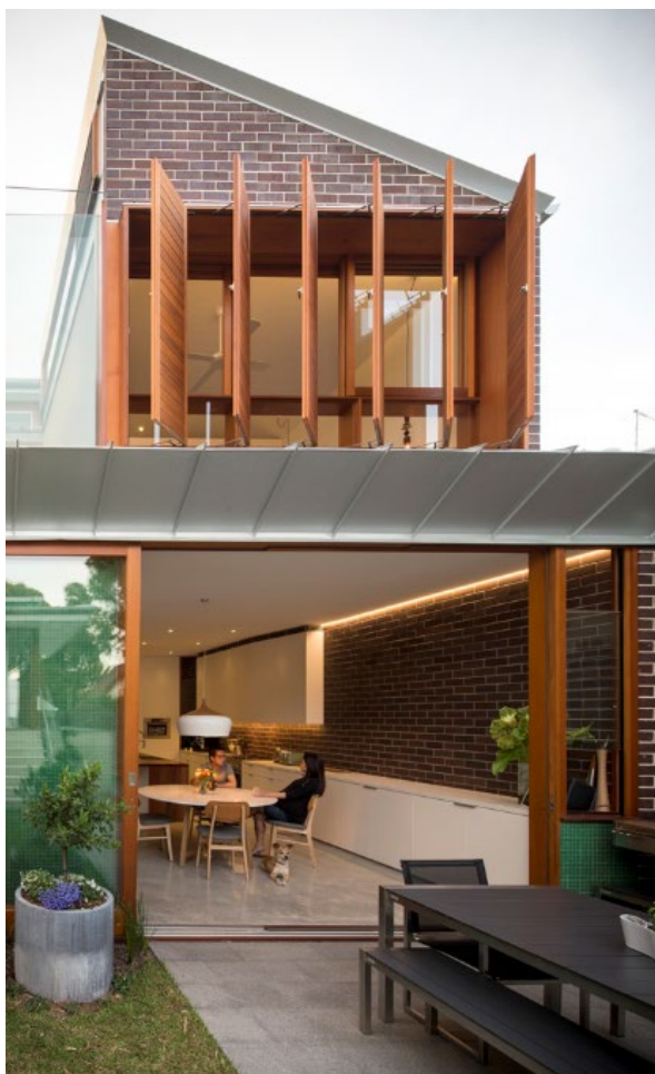
Figure 3-127 Adjustable screens allow control of sunlight
