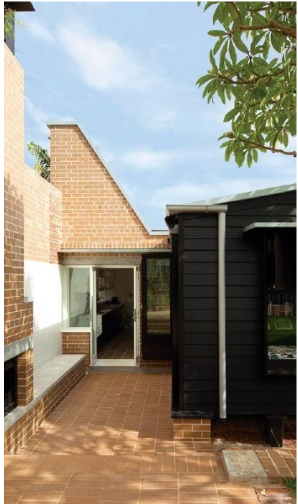
Figure 3-118 Brick patterns create visual interest and add detail and texture. Consider how facade and landscape treatments integrate into the overall design of the development
