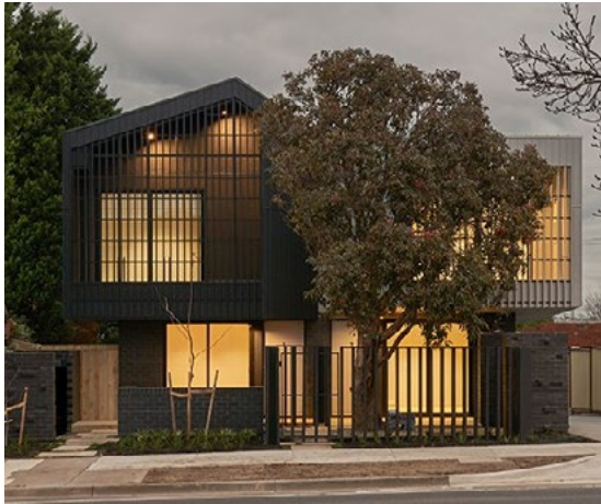
Figure 3-113 Example of transparent fencing landscaping in front setback and asymmetrical facade design
