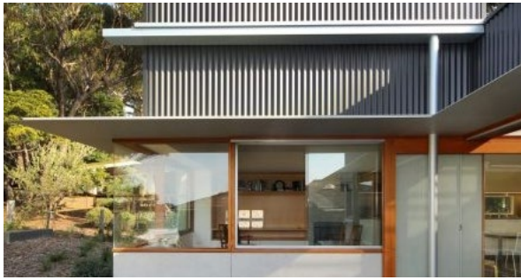
Figure 3-115 Awnings provide shelter and add articulation
