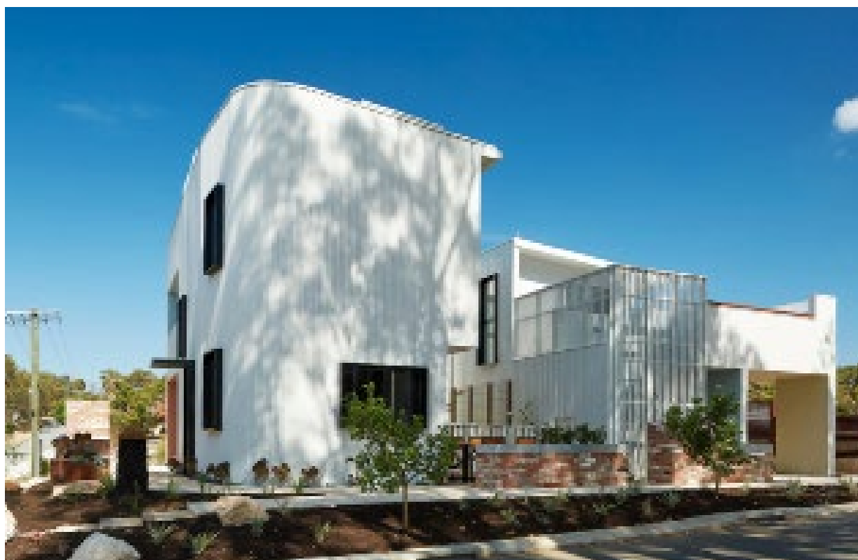
Figure 2-24 Manor House - 3 dwellings
