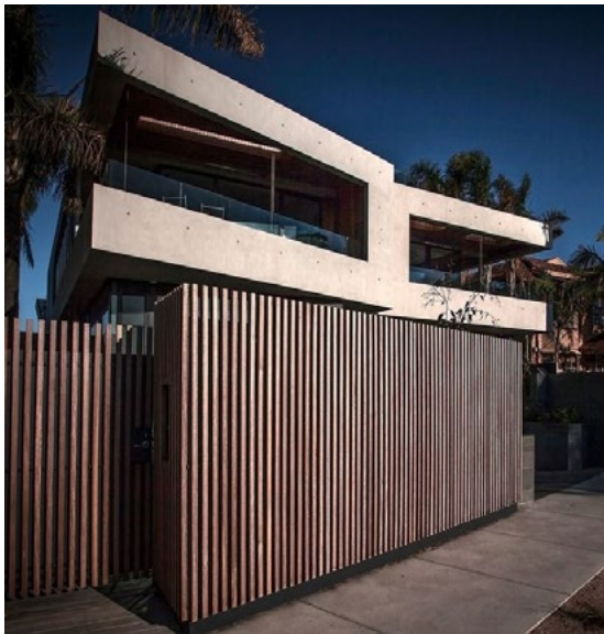
Figure 3-114 A combination of bold concrete and fine timber fencing create an interesting balance and contrast to the facade
