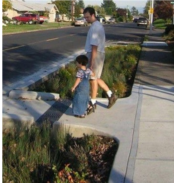
Figure 4-147 Rain gardens treat stormwater from the streets
