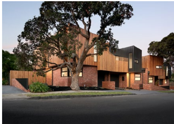
Figure 3-112 Varied building forms and a mixed palette of materials adds interest to the streetscape
