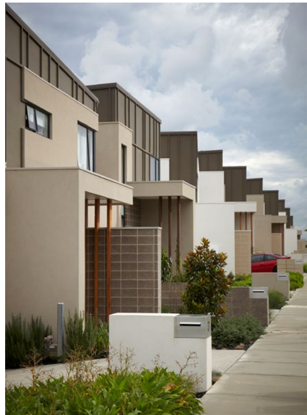
Figure 3-28 Landscaping softens the interface between the private and public domain
