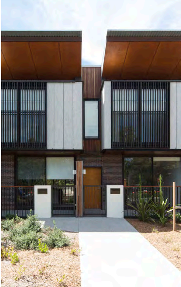
Figure 3-75 Living rooms setback from main circulation spaces by large landscape setback provides privacy
