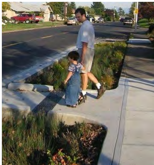
Figure 4-3 Rain gardens treat stormwater from the streets
