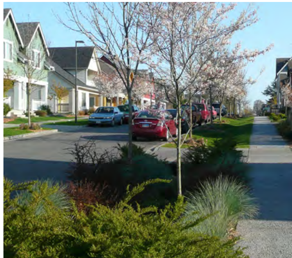
Figure 3-104 Swales can be attractive, and are able to filter and collect the stormwater
