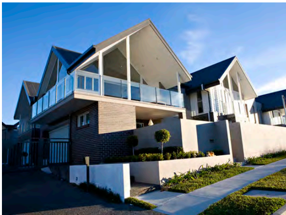
Figure 3-82 Roof form expressed
