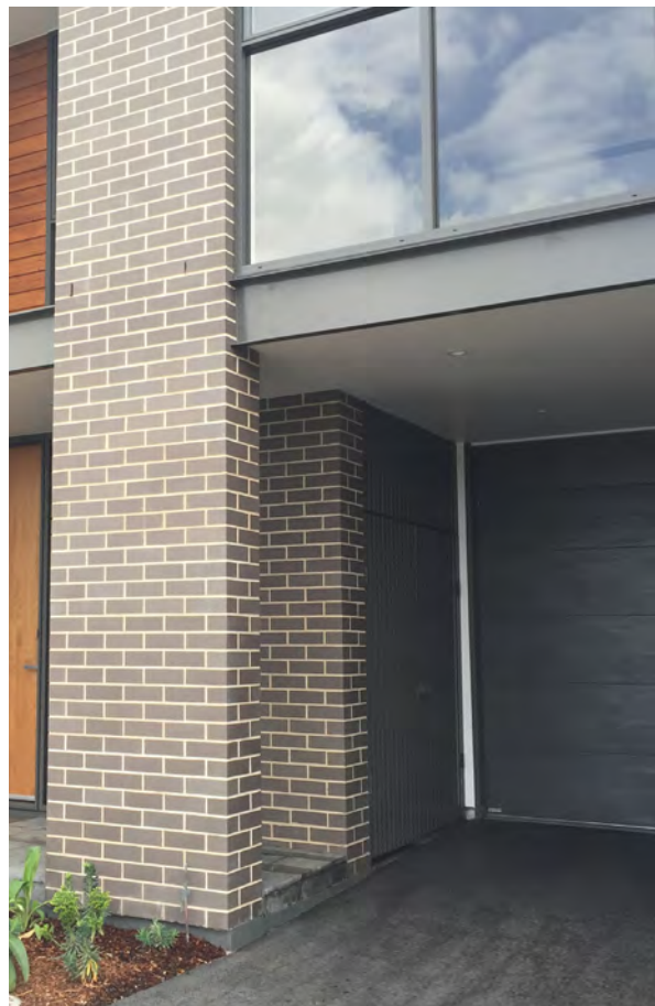
Figure 3-108 Provide bin areas that are screened and incorporated into the landscape or building design
