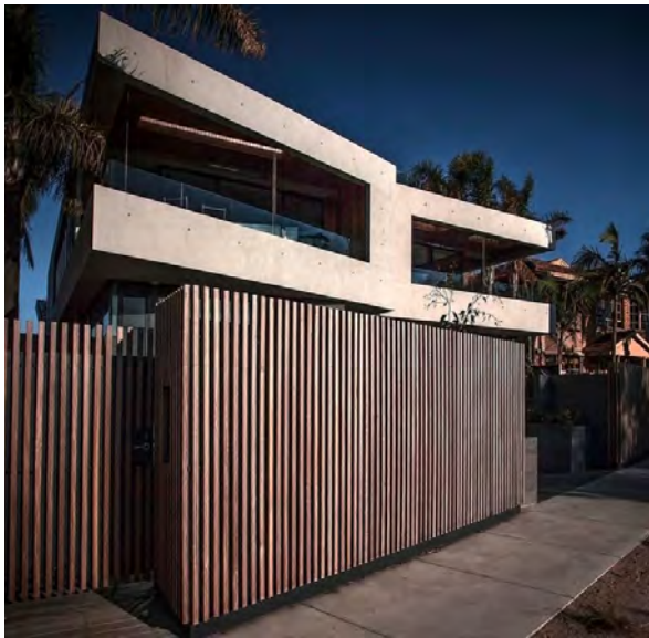
Figure 3-88 A combination of bold concrete and fine timber fencing create an interesting balance and contrast to the facade
