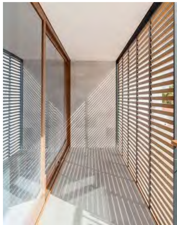
Figure 3-70 Fixed privacy screens can be used on balconies where there may be privacy concerns. Consideration should be given to how the screen is integrated into the facade
