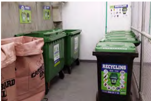
Figure 3-112 Waste and recycling areas should allow for sufficient space to manoeuvre bins and sort waste for recycling
