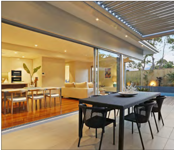
Figure 3-115 A universally designed dwelling provides step free door transitions and level flooring to reduce trip hazards
