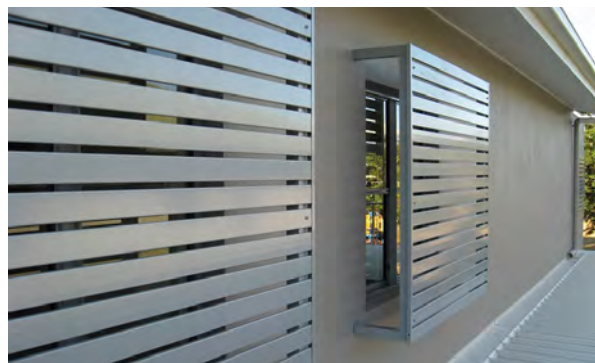
Figure 3-65 Poorly executed privacy screens. These block outlook, sunlight and daylight to windows and reduce amenity of room.
