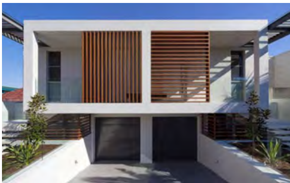
Figure 3-73 Privacy screens can be an integral part of the articulation. Changing the pattern and direction of the screen adds visual interest and asymmetry to the facade.
