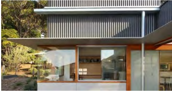
Figure 3-89 Awnings provide shelter and add articulation
