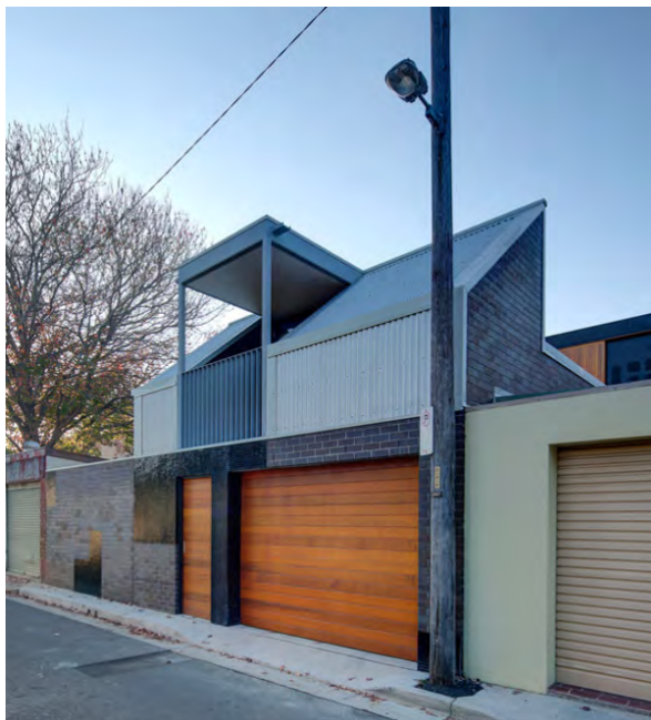
Figure 3-97 Rear outbuildings such as studios should be orientated to the lane to allow for passive surveillance and security
