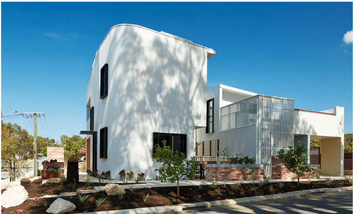
Figure 2.2-1 Manor House - 3 dwellings
