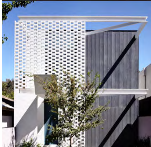
Figure 3-67 Privacy screens are integrated into the facade and provide part of the architectural expression
