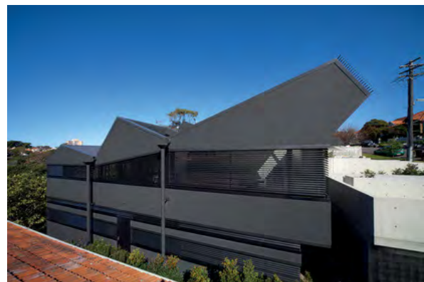
Figure 3-80 Interesting roof forms and integration of privacy and sun control devices to overall building design
