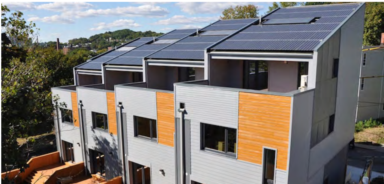
Figure 3-98 Roof mounted photovoltaics should be integrated into the design of the dwelling
