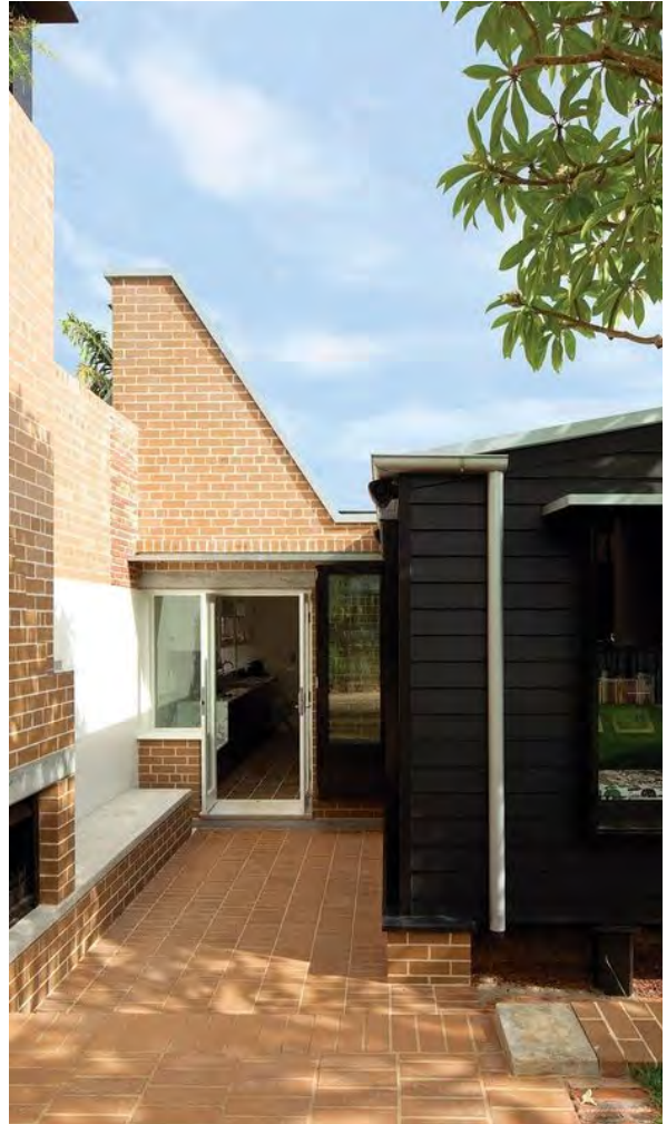
Figure 3-92 Brick patterns create visual interest and add detail and texture. Consider how facade and landscape treatments integrate into the overall design of the development
