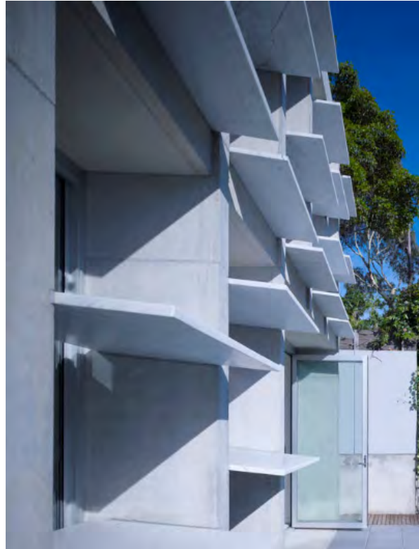
Figure 3-99 Light shelves can reflect sunlight deeper into rooms and provide shade from summer sun
