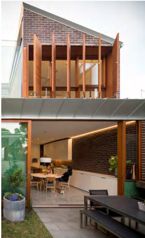
Figure 3-101 Adjustable screens allow control of sunlight
