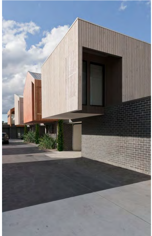
Figure 3-74 A poor acoustic outcome is achieved when driveways are in close proximity to bedrooms and living rooms, and driveways are hard paved reverberating sound.
