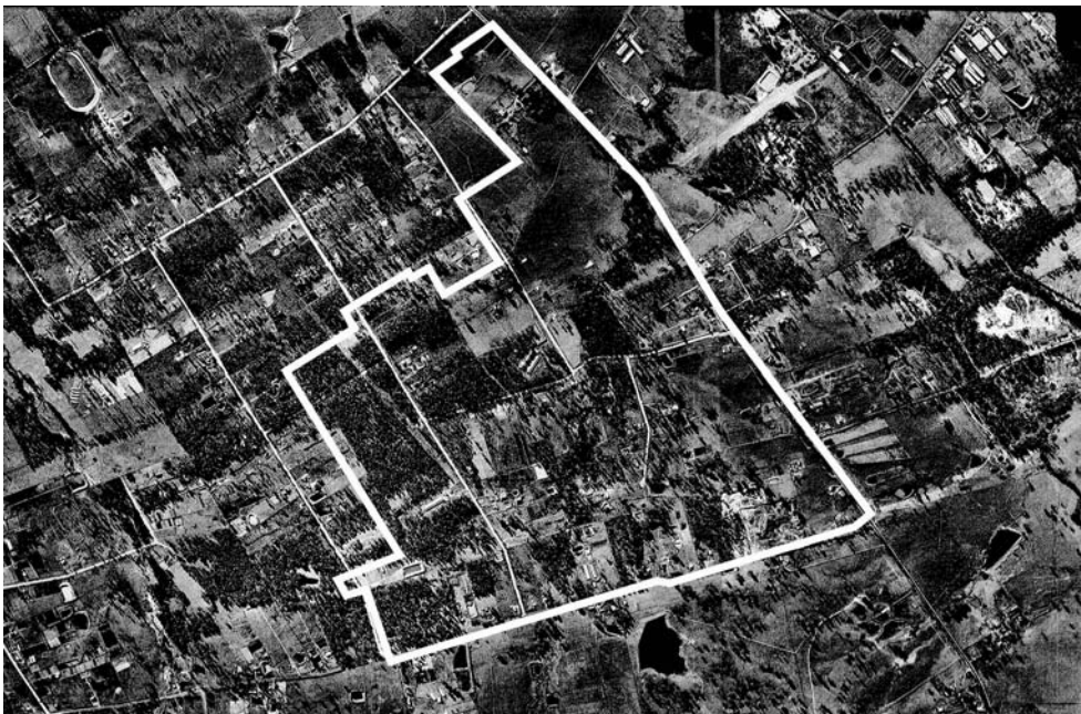
Figure 2.7 1970 aerial photograph of the Rouse Hill/Windsor Road area, showing the study area boundary (white line). Comparison to the photo in Figure 2.5 shows the development that has taken place since the first subdivisions of the Rouse Hill Estate in the 1950s. Small-scale rural development now dominates the area fronting Windsor, Cudgegong, Tallawong and Schofields Roads. (Source: Department of Lands NSW)
