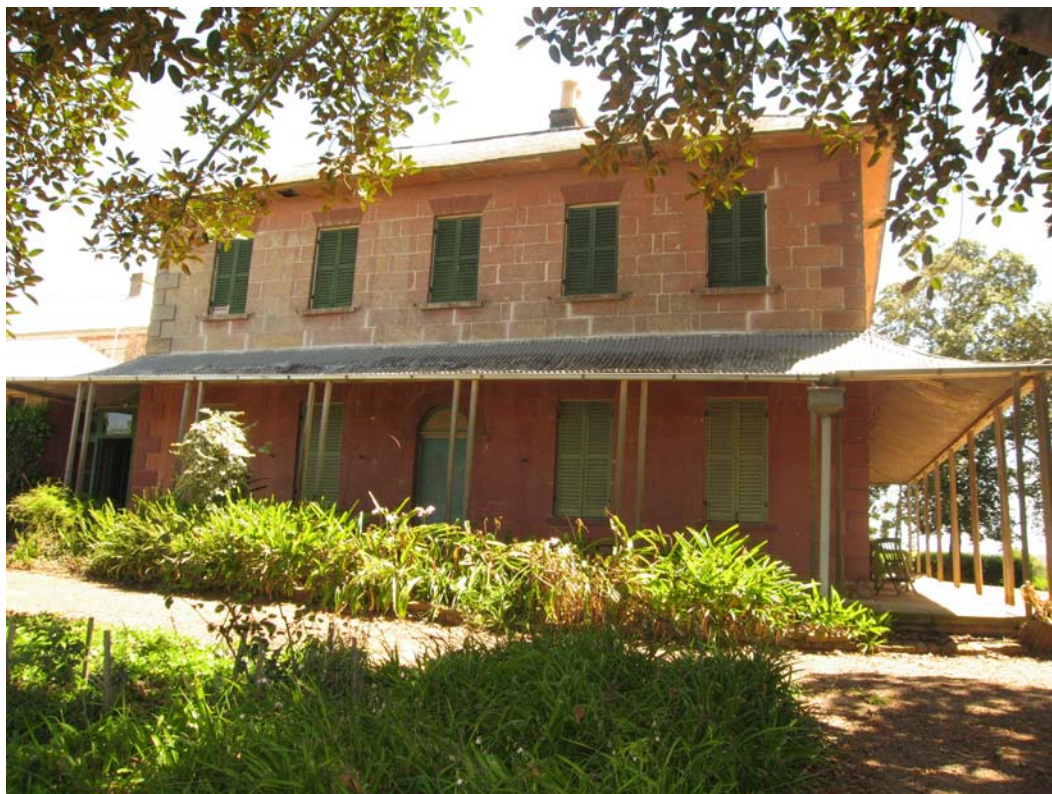
Figure 3.2 View of the south-facing elevation of Rouse Hill House, which is located within the study area. (Source: GML 2009)
