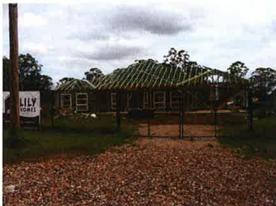
Figure 4.38 House under construction.
