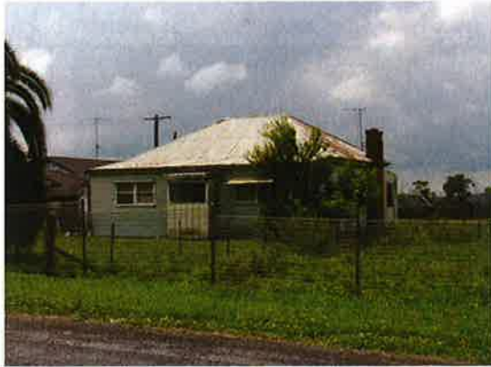
Figure 4.24 Weatherboard house at 45 Gurner Avenue.
