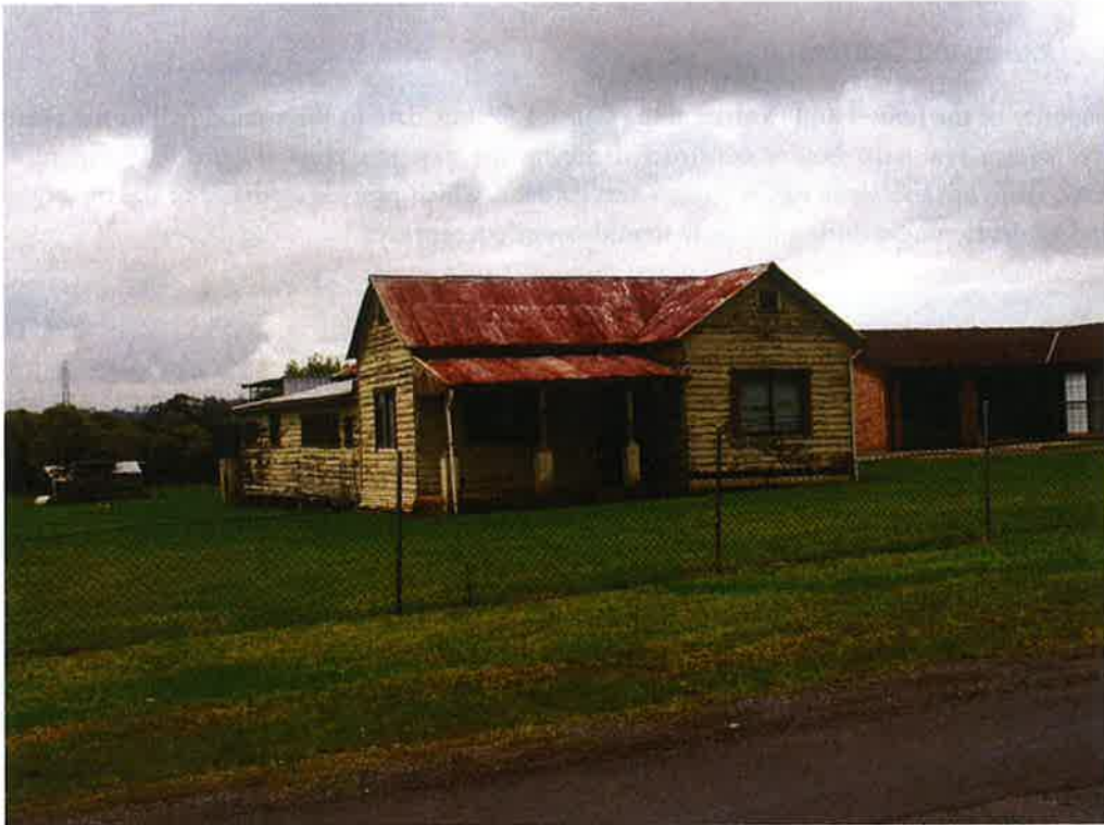
Figure 4.21 Weatherboard house at 11 Gurner Avenue.
