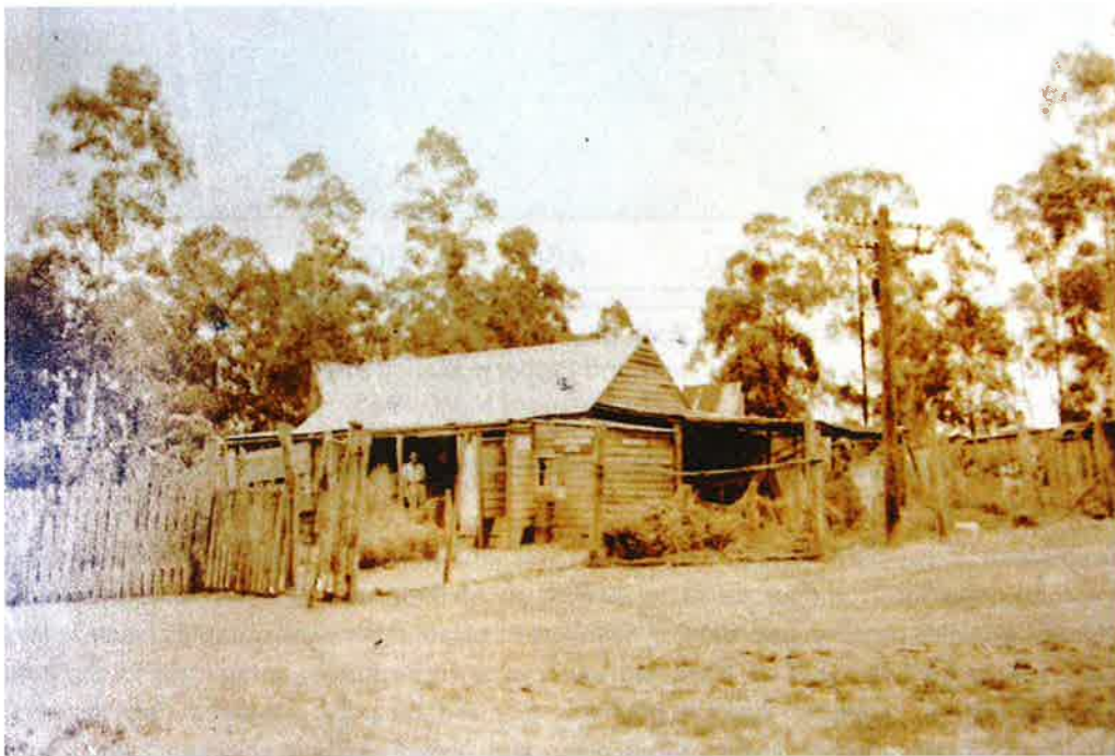
Figure 3.19 Austral post office, Tenth Avenue, c.1942 (Source: Erica Clarke).
