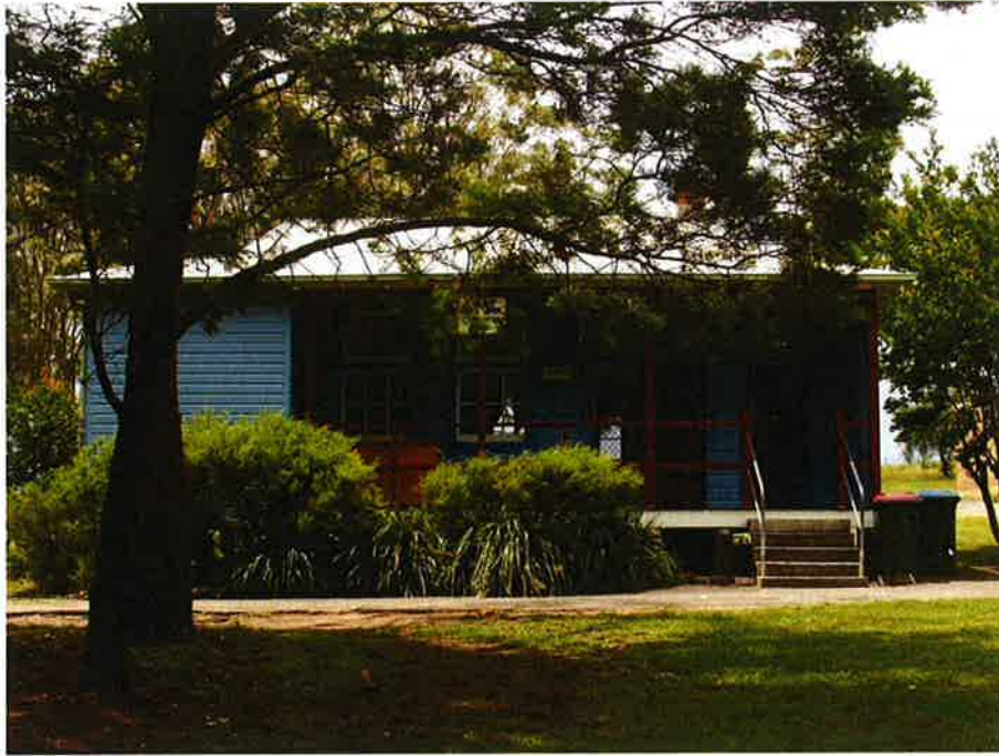
Figure 4.94 Original 1923 timber school building, Leppington Public School.
