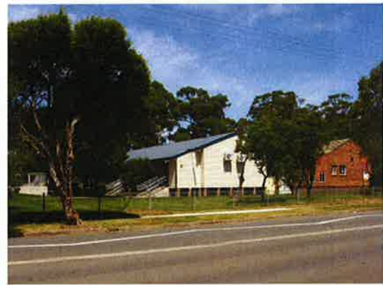
Figure 4.63 Austral Public School, 1950s fixed timber building.
