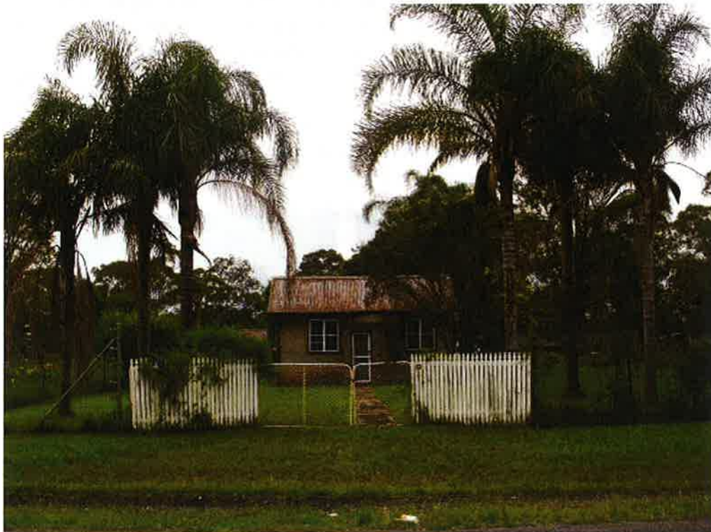
Figure 4.59 Cement rendered worker's cottage at 60 Fifth Avenue (40 Browns Road).
