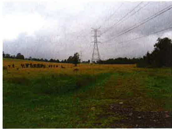
Figure 4.7 Transmission lines crossing the paddocks east of Kemps Creek Substation.
