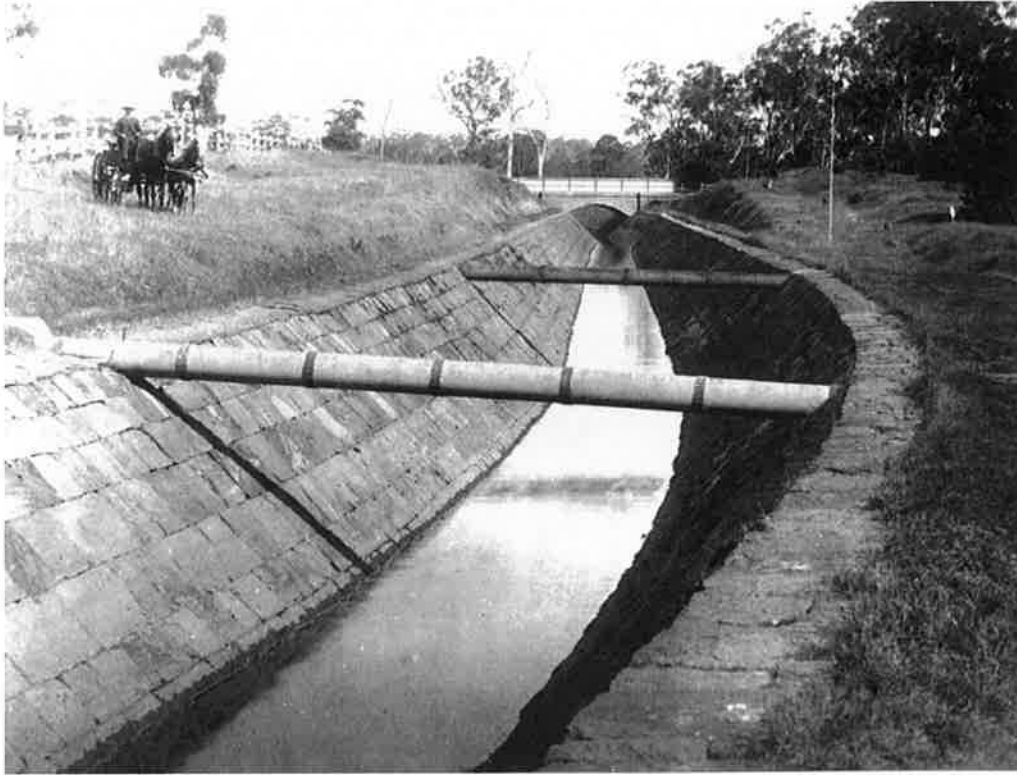
Figure 3.23 A section of V-shaped masonry Canal at 24 1/2 miles, with the original Raby Road bridge in the background (Section 6, Inventory 48). Although this section of the Canal is south of the study area, the image illustrates similar forms of construction to those used in the study area (Source: Edward Higginbotham & Associates 2002:37; from Sydney Water/SCA Historical Research and Archives Facility, Ref: X841025-8).
