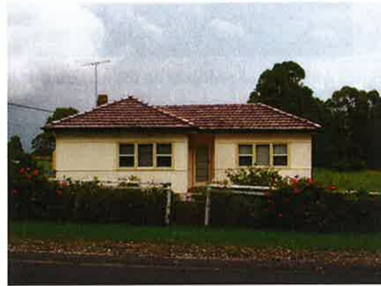
Figure 4.90 Mid-twentieth century house on Rickard Road.
