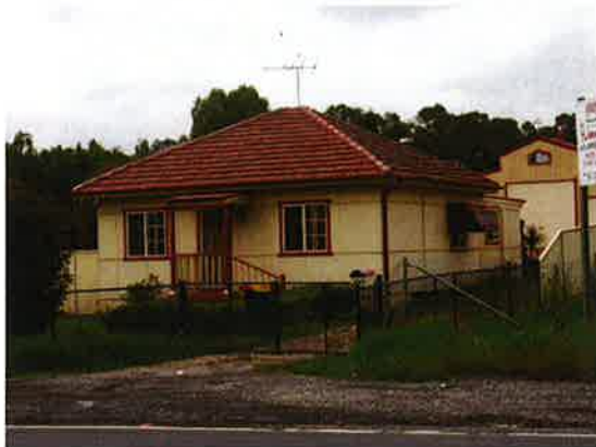
Figure 4.52 Fibro clad house at 280 Fifteenth Avenue.
