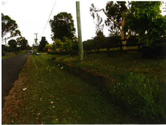
Figure 4.77 Low retaining wall built of squared sandstone blocks, 46 Kelly Street.
