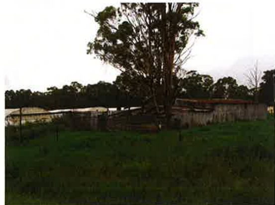
Figure 4.18 Farm buildings to the rear of 85 Gurner Avenue.
