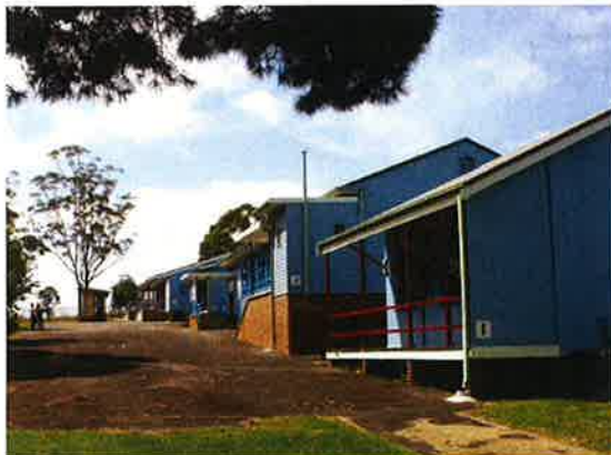
Figure 4.95 Row of timber demountables, Leppington Public School.
