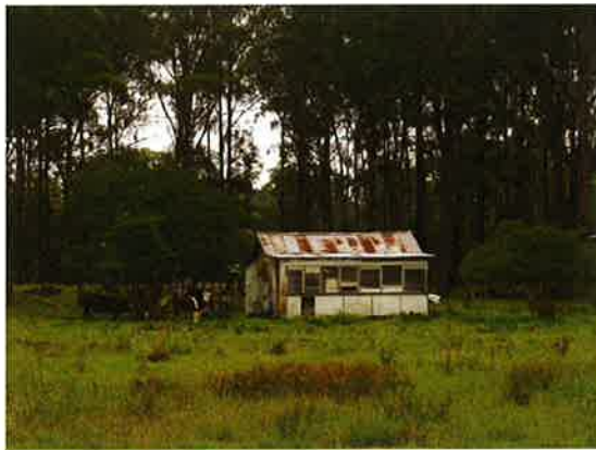
Figure 4.79 Small, dilapidated hut at 1 Kelly Street.
