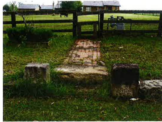
Figure 4.78 Sandstone step and retaining wall, 46 Kelly Street.
