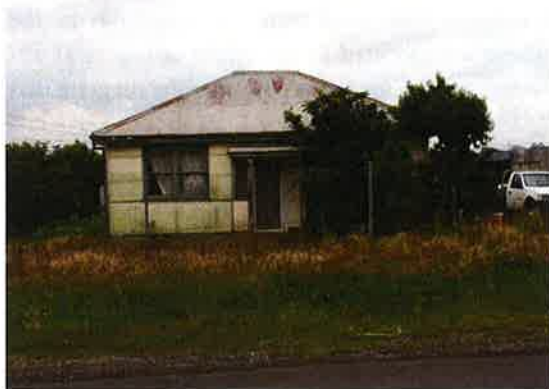
Figure 4.22 Fibro house at 15 Gurner Avenue.
