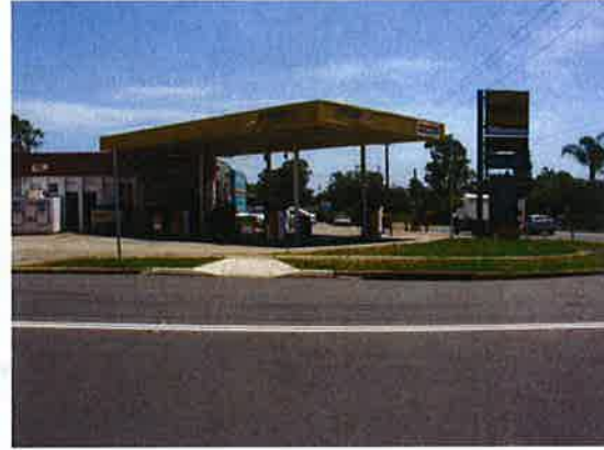
Figure 4.41 Speedway petrol station at the junction of Edmondson and Fifteenth Avenues.
