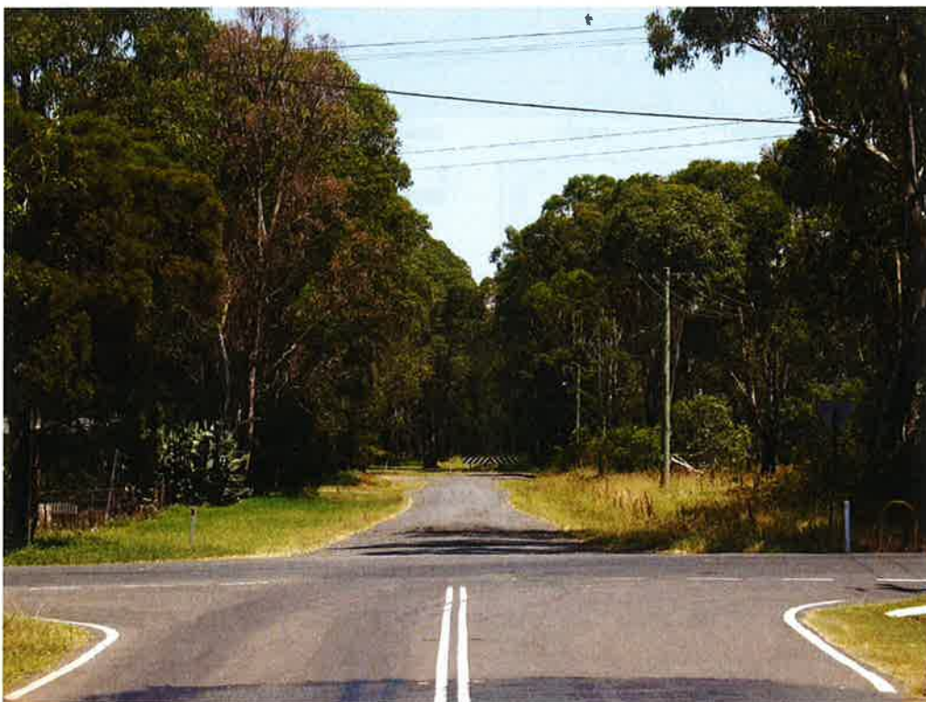
Figure 4.31 View along Seventh Avenue, to the west. Seventh Avenue is interrupted between Edmondson and Fourth Avenues by the alignment of a local creek.
