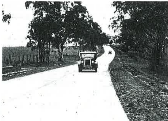
Figure 3.14 After reconstruction: Completed concrete pavement between Carne's Hill and Narellan, 1 ½ miles south of the water-race. (Source: Hall 1931:89).
