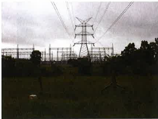
Figure 4.6 Kemps Creek Substation.
