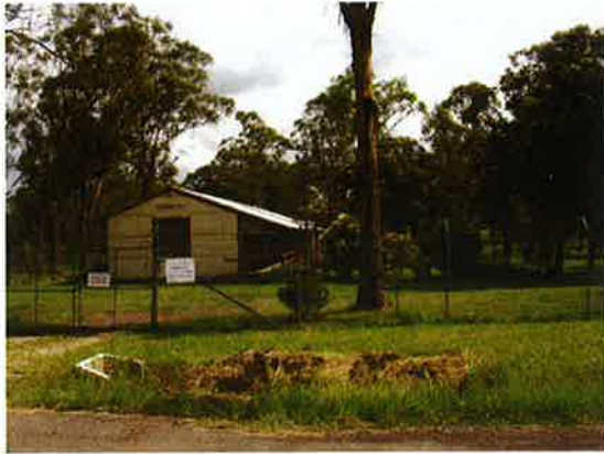
Figure 4.64 Camp Austral, view from the south.
