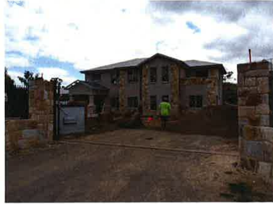
Figure 5.202 Child care centre under construction.
