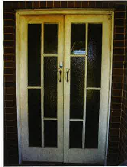
Figure 5.144 Detail of glass-panelled French doors.
