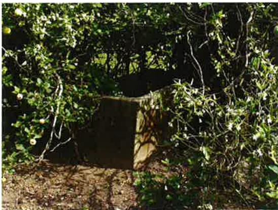
Figure 5.64 Concrete trough, overgrown by a flowering quince.
