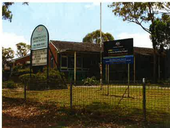
Figure 5.100 Northern group of school buildings; view from Rickard Road.
