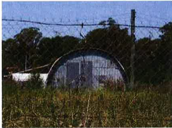
Figure 5.170 North elevation of the Nissen hut on the corner of Seventh and Edmondson Avenues.
