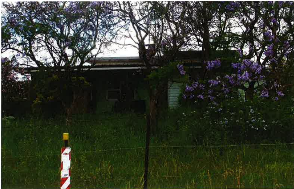
Figure 5.84 Front of dwelling, 1720 Camden Valley Way.
