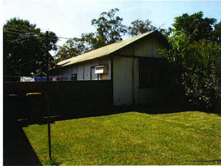
Figure 5.146 Former feed shed, to the rear of the house.
