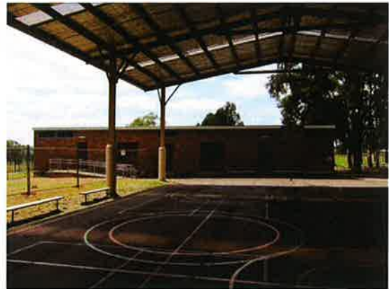
Figure 5.118 Building C and sports court.
