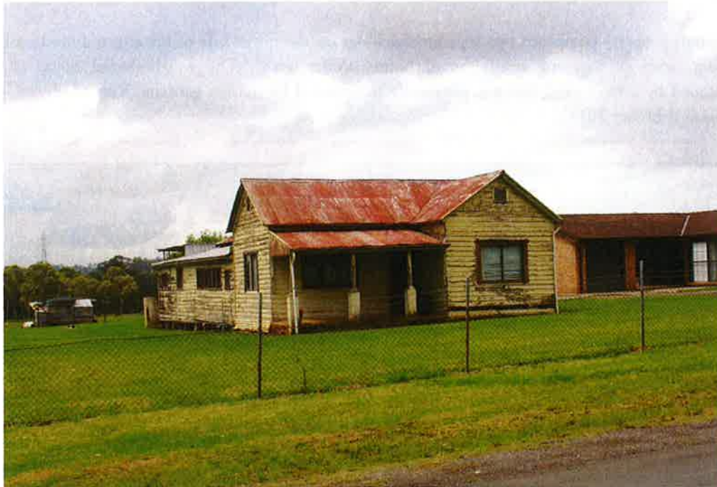
Figure 5.197 Weatherboard house at 11 Gurner Avenue, view from the southwest.
