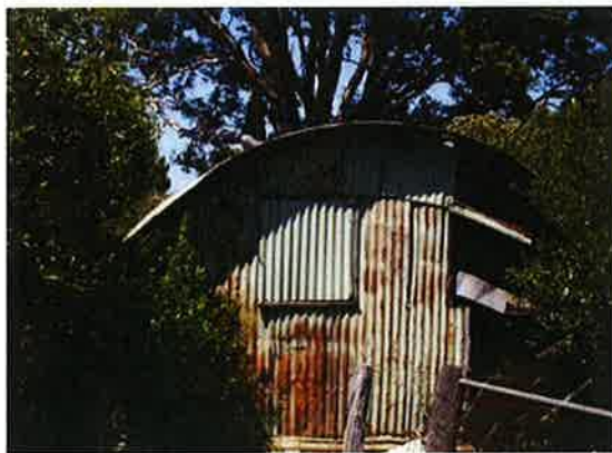
Figure 5.172 Nissen hut on Bringelly Road; view of the west elevation with original cladding and windows.
