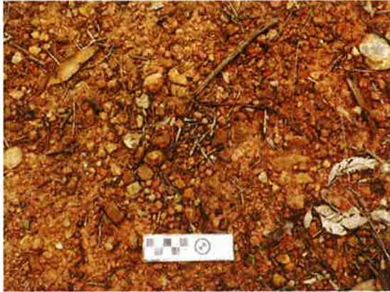
Figure 5.179 Compacted clay and gravel surface, exposed in unused area of road reserve, on the east side the Canal.
