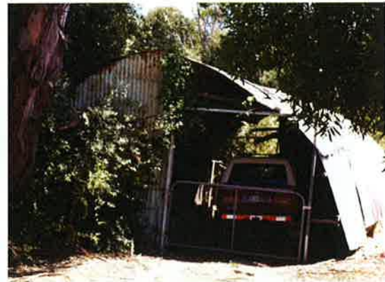
Figure 5.173 Nissen hut on Bringelly Road; the east end has been modified to provide parking access.
