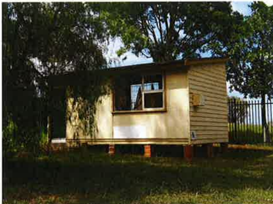
Figure 5.113 Weather shed (Building N).
