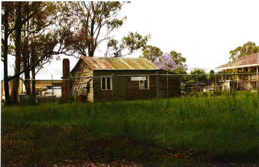
Figure 5.195 The house at 15 Seventeenth Avenue.
