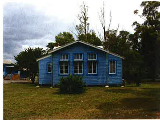
Figure 5.104 Rear of original Raby Public School building; view from the southeast.
