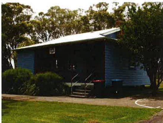
Figure 5.103 Original Raby Public School building, 2011; view from the west
