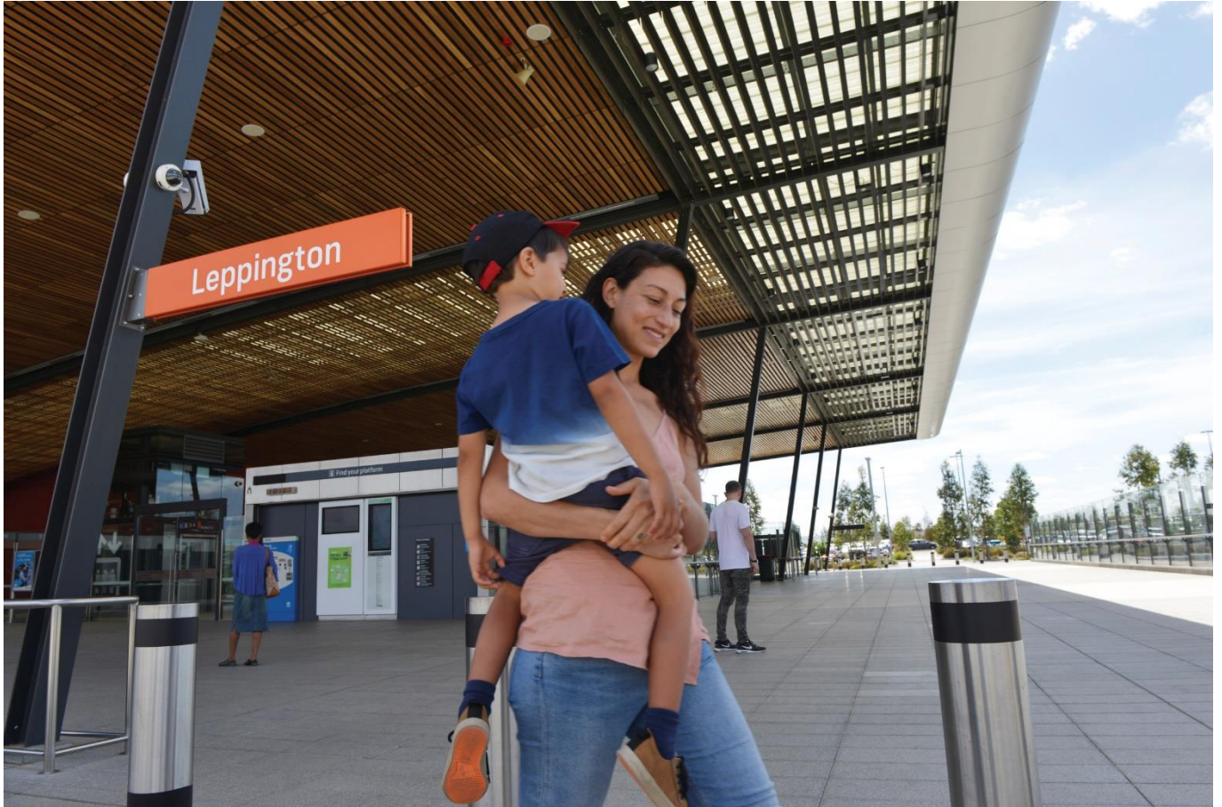
Leppington Railway Station was opened 2015, courtesy: Adam Hollingworth, DPE.
