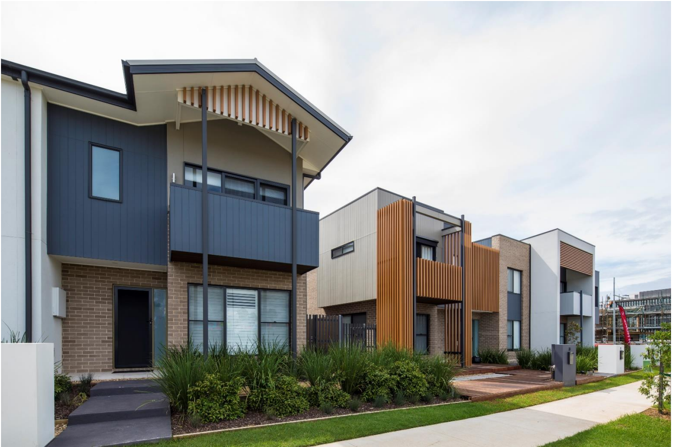
New housing in the South West Growth Area, courtesy: Greenfields Development Company.
