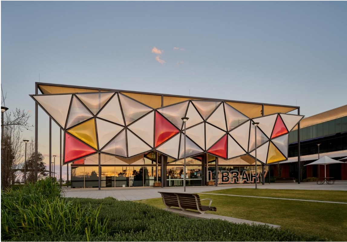
Oran Park Library opened 2018, courtesy: Greenfields Development Company.
