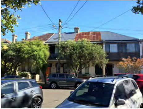
Figure 14 — View of terraced building on southern side of Silver Street (Part of Group B)
