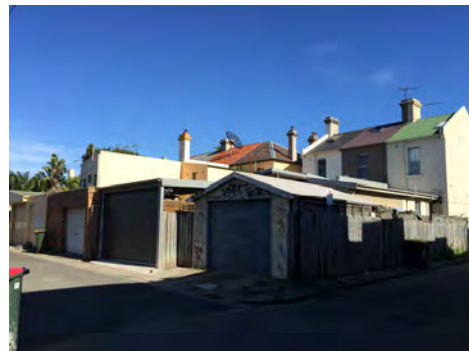
Figure 17 — Rear view of the two storey terraces
