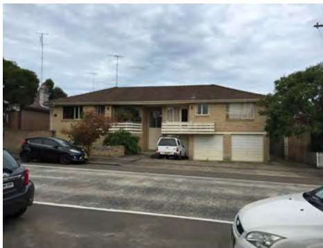
Figure 58 — View of later residence on the eastern side of Wardell Street
