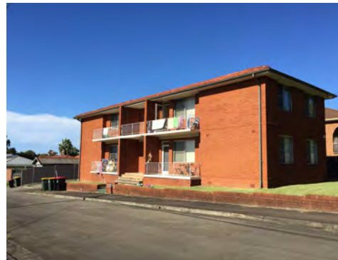
Figure 84 — View of a later red brick apartment block
