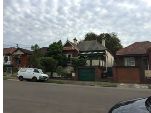
Figure 47 — Two sites that have been modified to include a small garage
