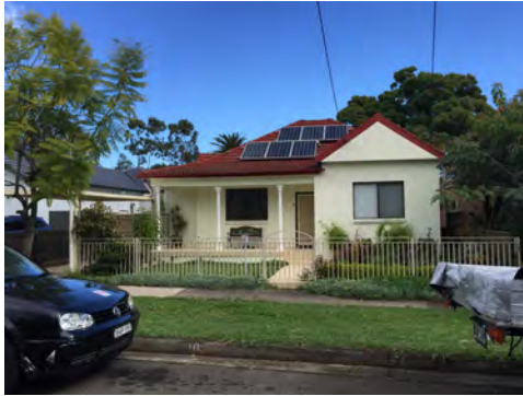
Figure 85 — A heavily modified Federation cottage
