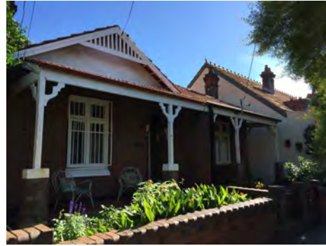
Figure 21 – View of where the Group C and Group D houses adjoin
