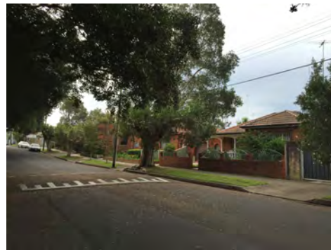
Figure 61 — View of modifications to later houses on Riverside Crescent
