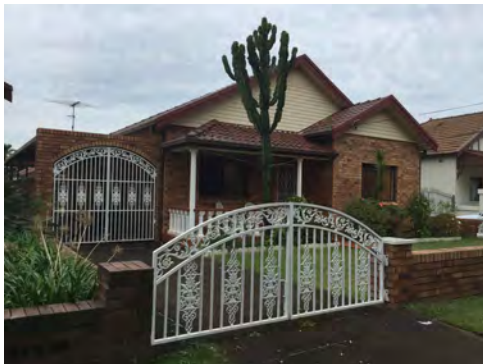
Figure 73 — Modified example of a Pre WW1 dwelling in Acacia Street
