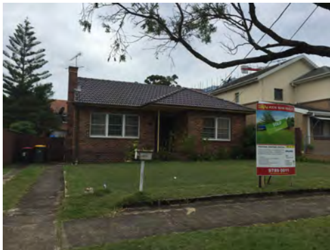
Figure 83 — Example of a post 1943 dwelling
