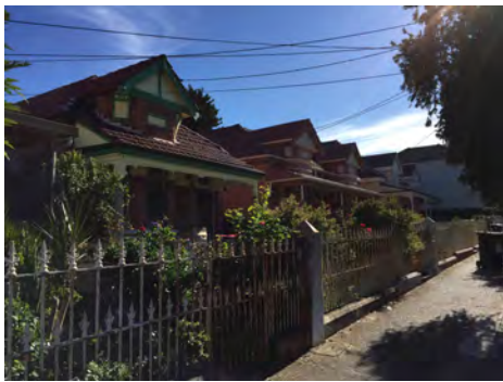
Figure 18 — View of Group A houses
