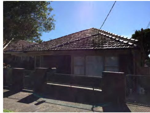
Figure 7 — North side of Church Street – Group C Building
