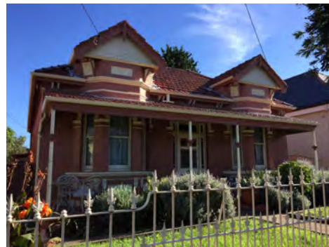
Figure 19 — Detail of the symmetrical facade
