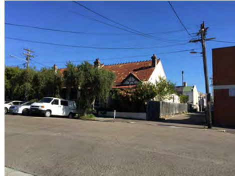
Figure 15 — View of end terrace of Group C buildings on Gladstone Street
