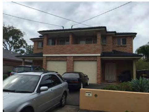
Figure 88 — A recent two storey semi detached dwelling
