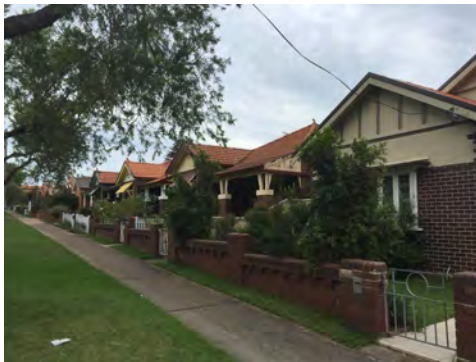
Figure 81 — Looking north along Cleary Street at the Group A buildings
