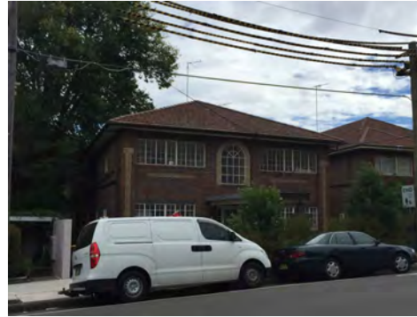
Figure 57 — View of the easternmost Inter-war apartment block in Group A
