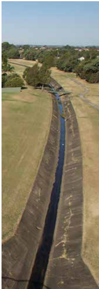
The existing concrete stormwater channel.
