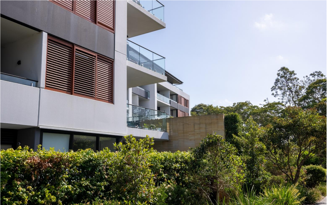
Figure 1: Residential flat building in Lane Cove
