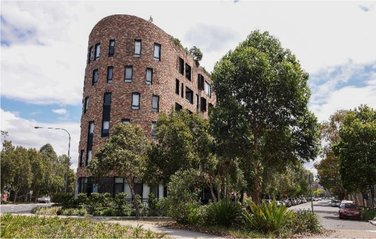
Figure 4: Residential flat building on Huntley Street, Alexandria
