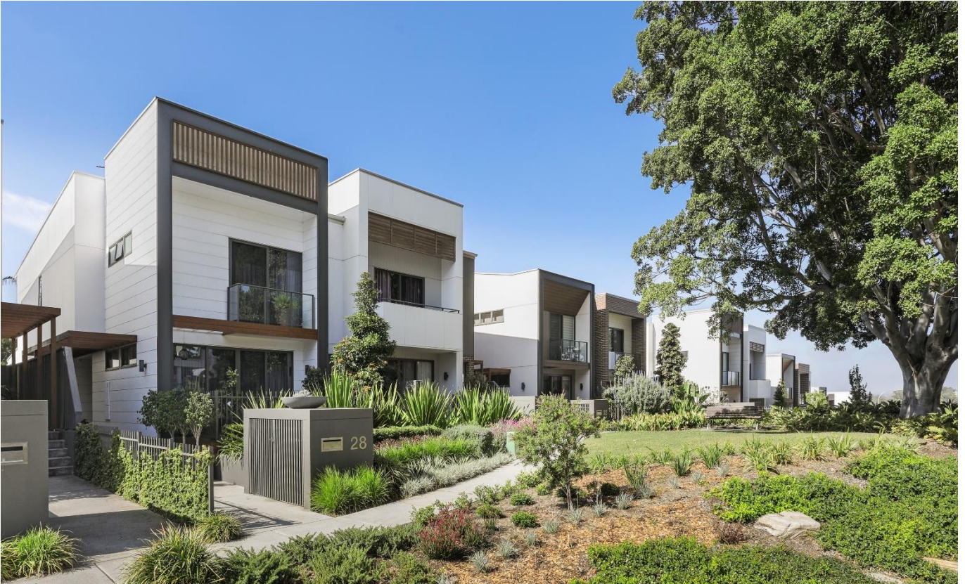
Figure 12: Dual occupancy housing in Ryde
