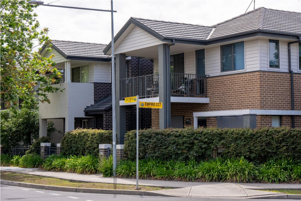
Figure 9: Manor house in Thornton
