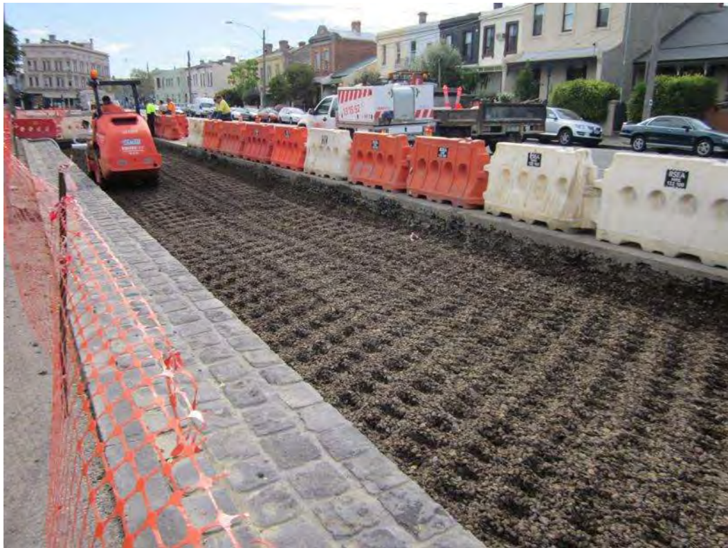
City of Melbourne - http://urbanwater.melbourne.vic.gov.au/projects/permeability-infiltration/eades-place-permeable-parking/
