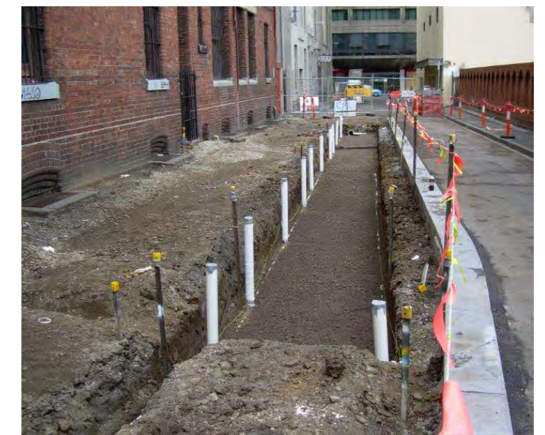
Godfrey St Infiltration trench under construction Source: http://urbanwater.melbourne.vic.gov.au/projects/greening-projects/godfrey-street-greening-project/
