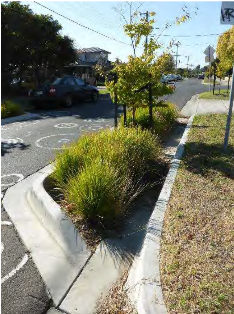
Figure 7 - Example of a street tree passively irrigated from the surface by road runoff (E2Designlab)
