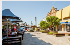
High quality paving to improve traffic flow and provide seamless pedestrian movement
