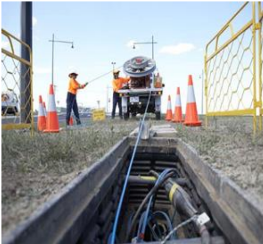
Figure 11 Cable being inserted into duct
