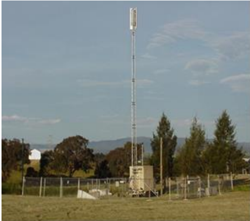
Figure 12 Temporary macrocell base station (2 panel antennas) on lattice support mount.
