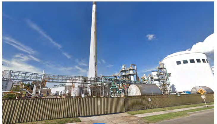
Figure 9: Ixom's sulfuric acid storage tanks along Foreshore Road
