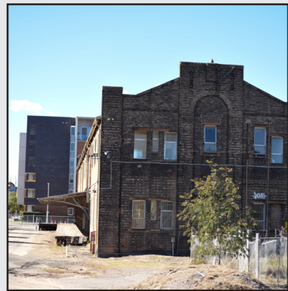
Paint Shop building.
