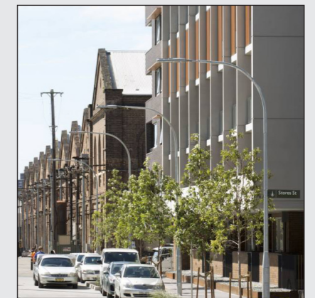
Platform Apartments at North Eveleigh.
