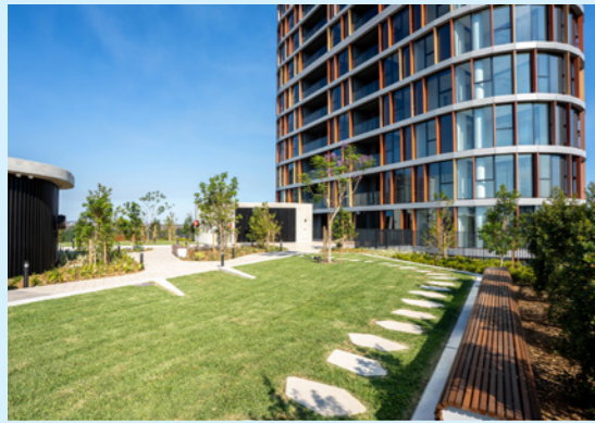
Shared amenity A communal roof deck has shared facilities like barbecues and covered dining areas. A skylight in the centre lights an atrium to the offices. Images: Tom Roe, Mike Chorley.
