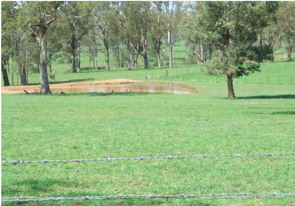
Photograph 8: Farm dams are constructed of locally won material
