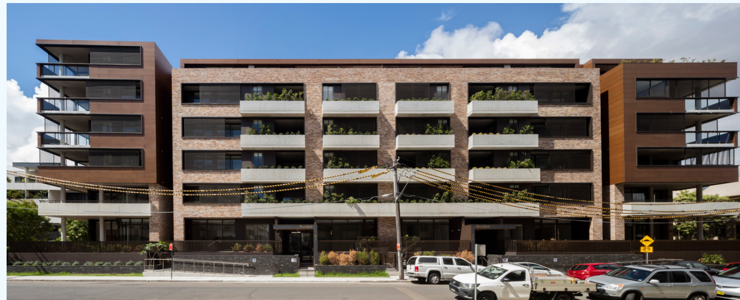
Mediating the levels The 3-m landscaped setback to all street edges allows universal access, private entries and planting for privacy to be incorporated. Image: Brett Boardman Photography.
