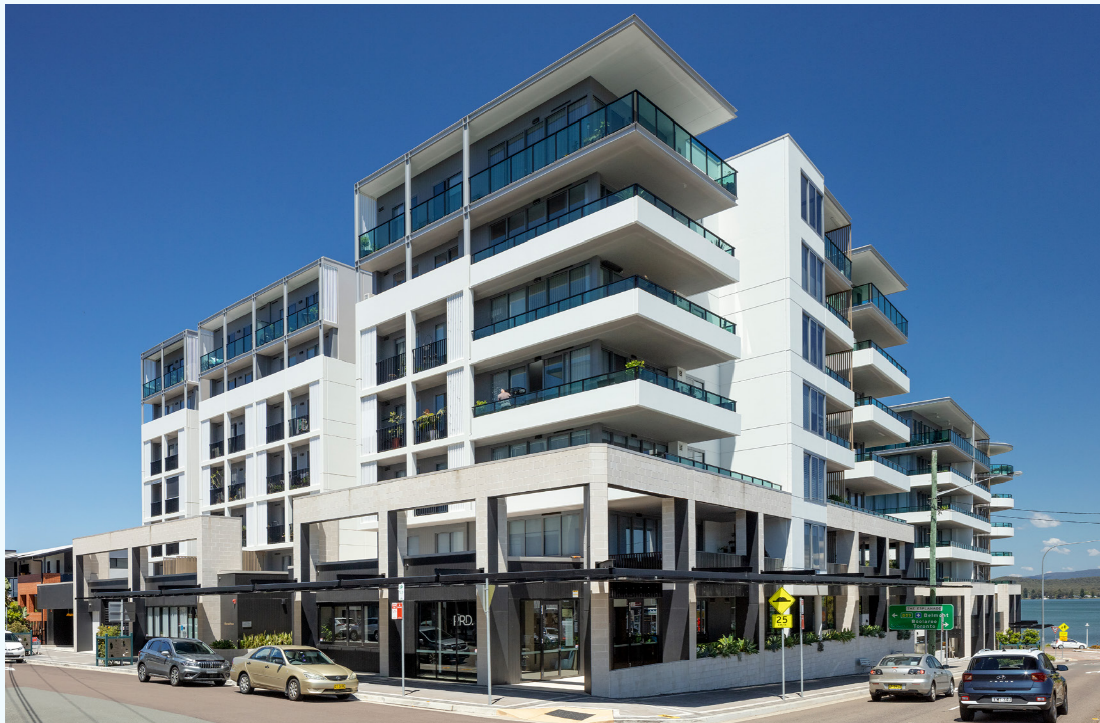
Living by the lake Generous apartments with high levels of amenity overlooking Lake Macquarie, viewed from the north-east corner of the site. All photos: Simon Wood Photography.
