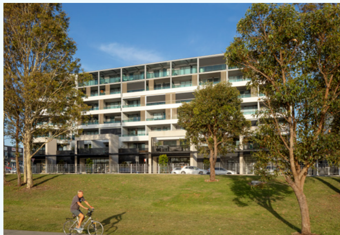
Base, middle, top View from lakeside reserve.
