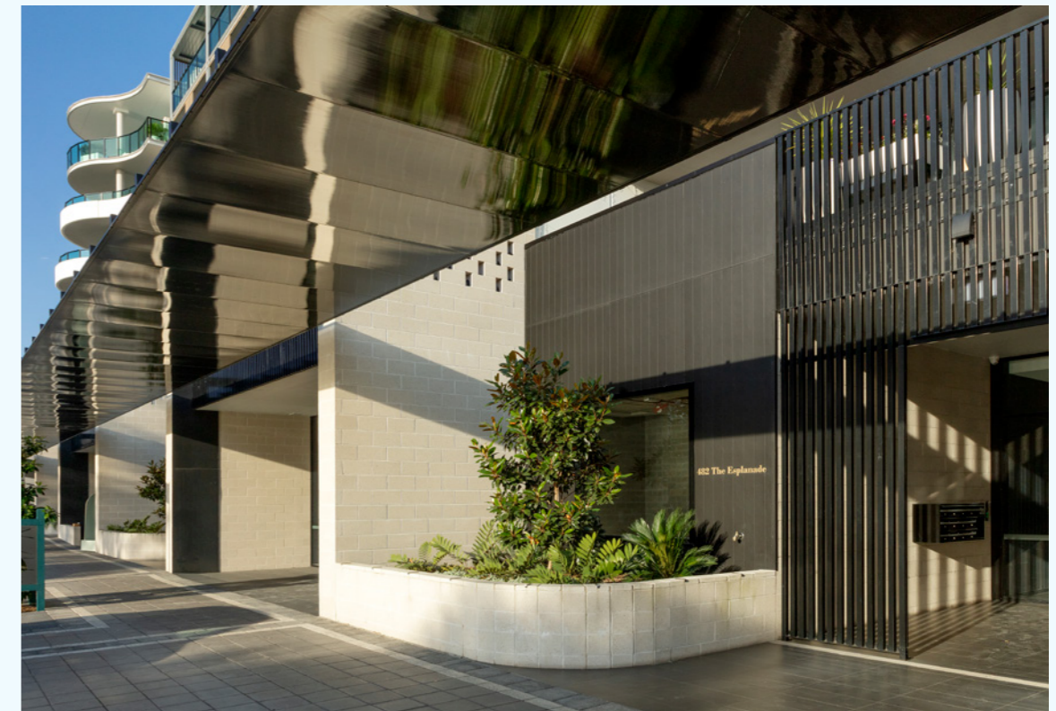
Blockwork portals The street awning is articulated as a separate element in the building. Residential entries are defined between the retail tenancies with landscaping and varying materials.
