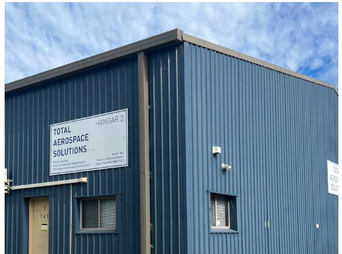
A hangar operated by Total Aerospace Solutions.
