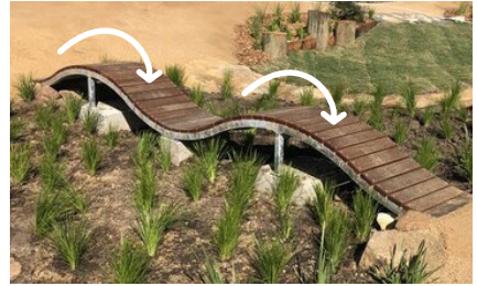
Double roller. A timber feature that consists of two rollers and allows the rider to 'pump' across.
