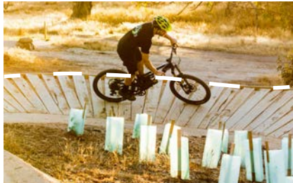
Berm. A berm is a banked corner in the track. They have an outer edge that runs the entire length of the corner to support the rider as they turn.
