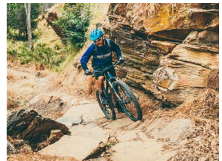
Trail armoured. Armoured is a method of using large rocks to pave a trail and prevent erosion.
