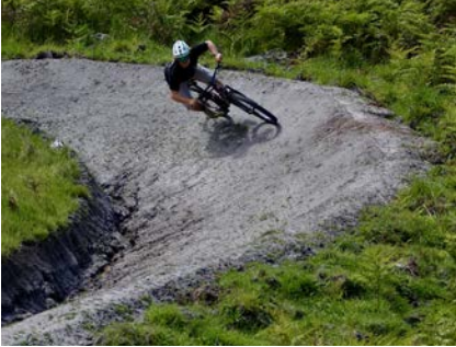
Berm corner. A bermed corner has a banked outer edge that runs the entire length of the corner to support the rider as they turn.
