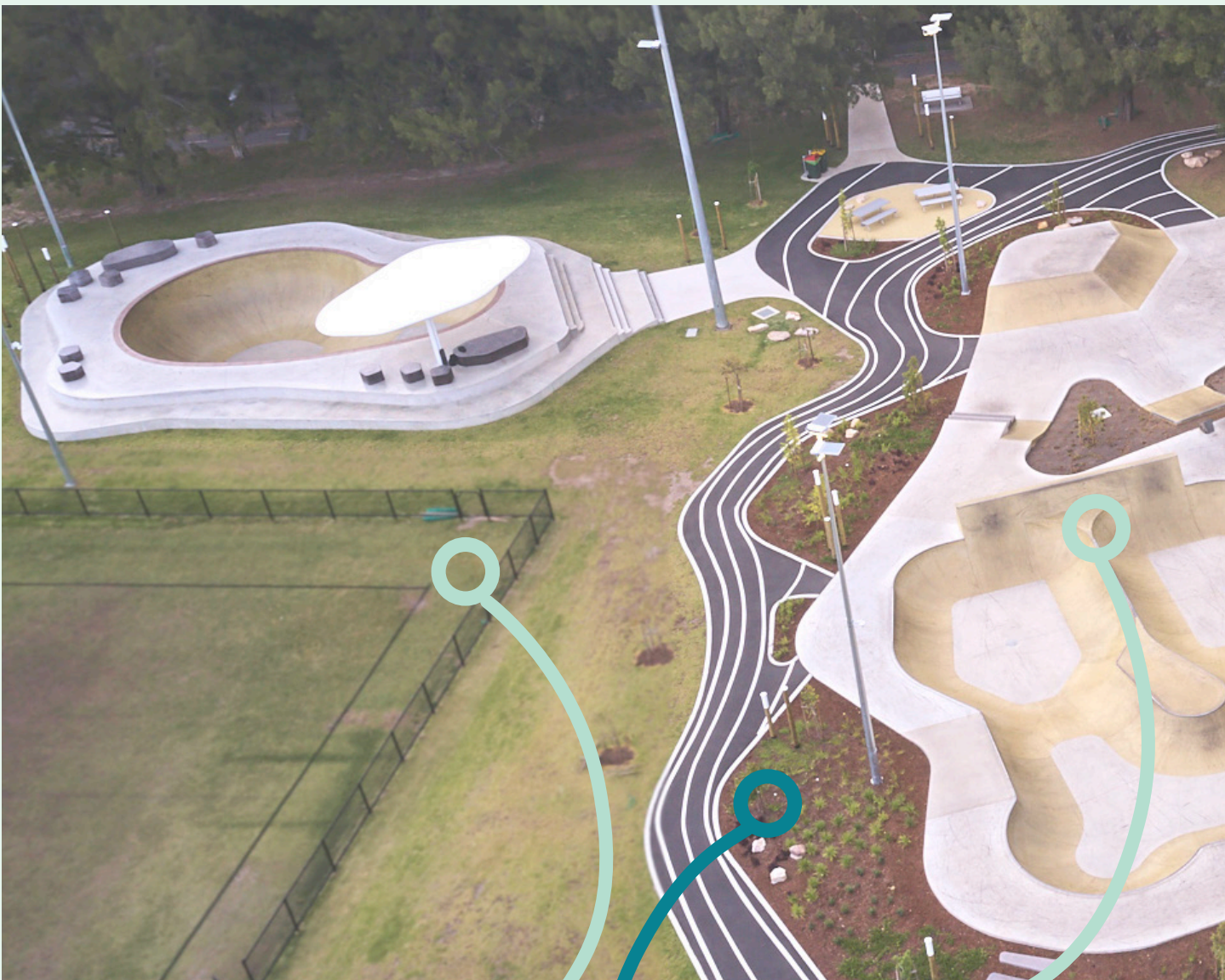
Amenities building. Located nearby to facilitate family use and provide convenience for users
