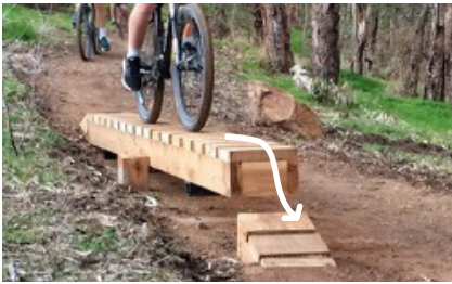
Drop. A feature with loss of elevation that allows the rider to lift off the track.
