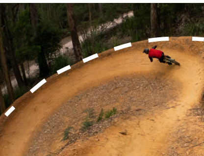
Rolling grade knicks. A knick is a semicircular, shaved down section of the trail, that is sloped to drain water.
