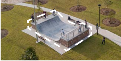
Mini ramp. A feature similar to a halfpipe, but has a smaller overall size and less steep transitions.
