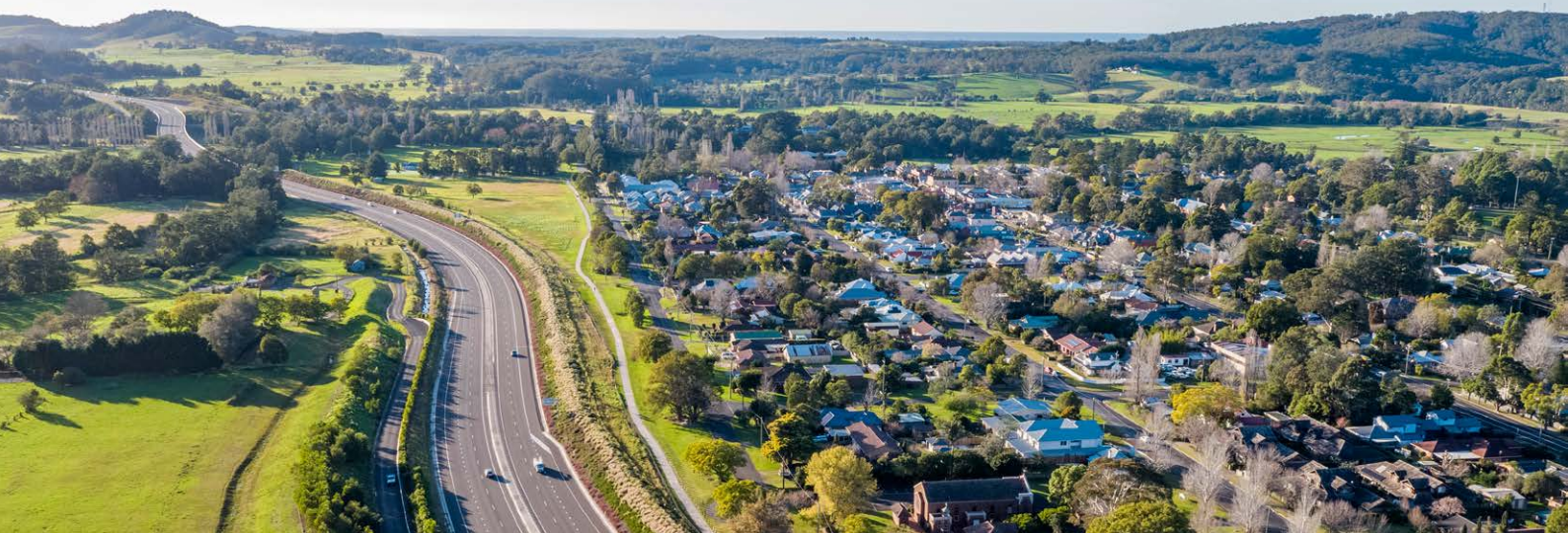
The Berry Bypass, Shoalhaven, NSW
