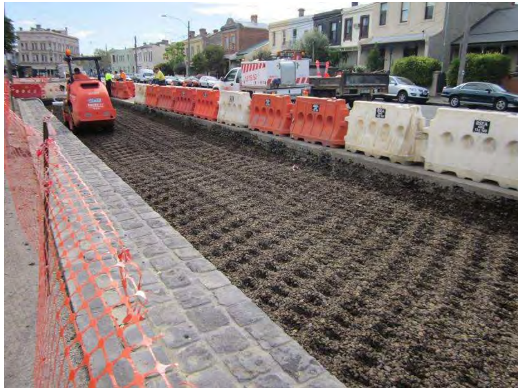
City of Melbourne - http://urbanwater.melbourne.vic.gov.au/projects/permeability-infiltration/eades-place-permeable-parking/
