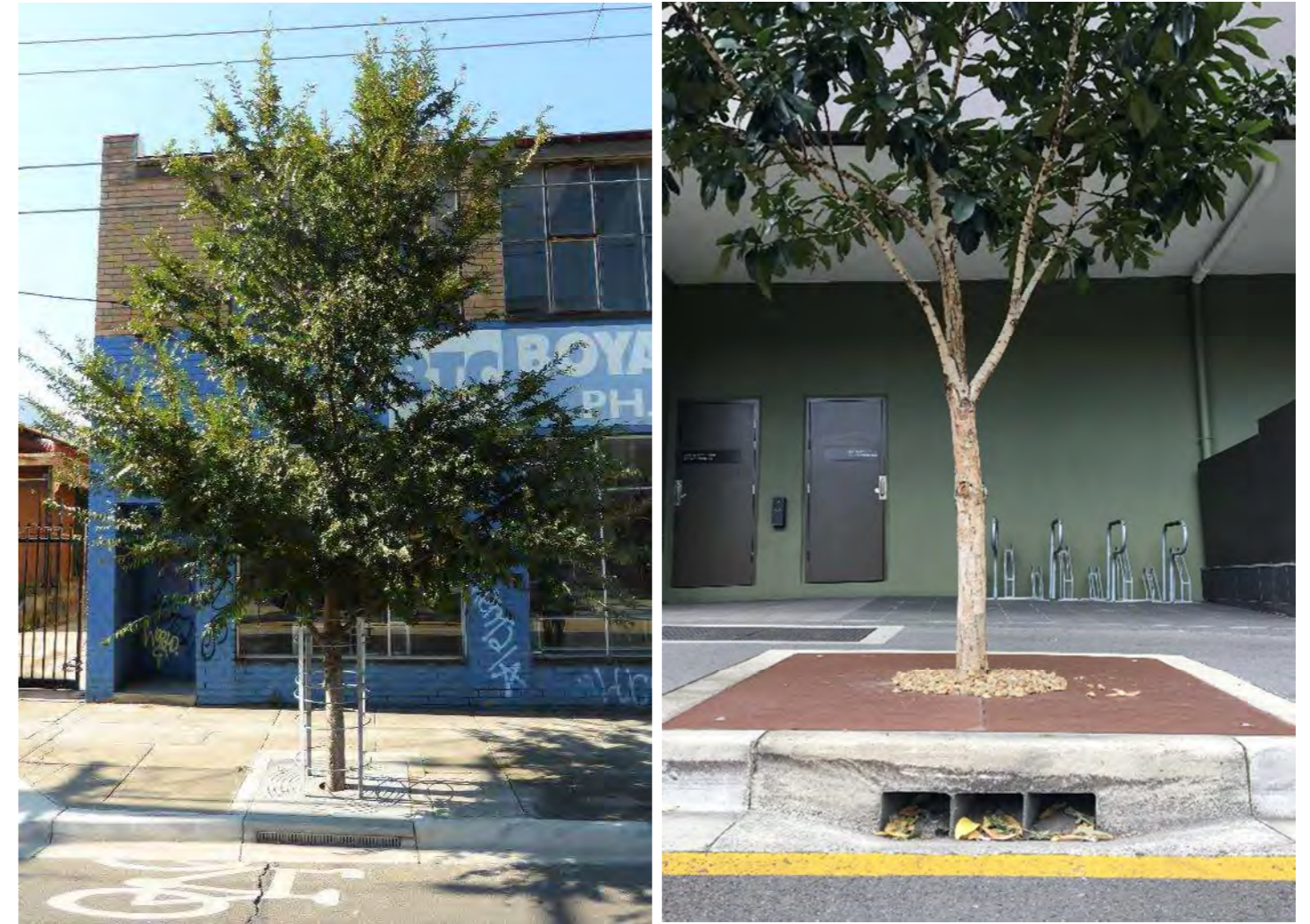
Example images of grated tree pits in Victoria (E2Designlab)
