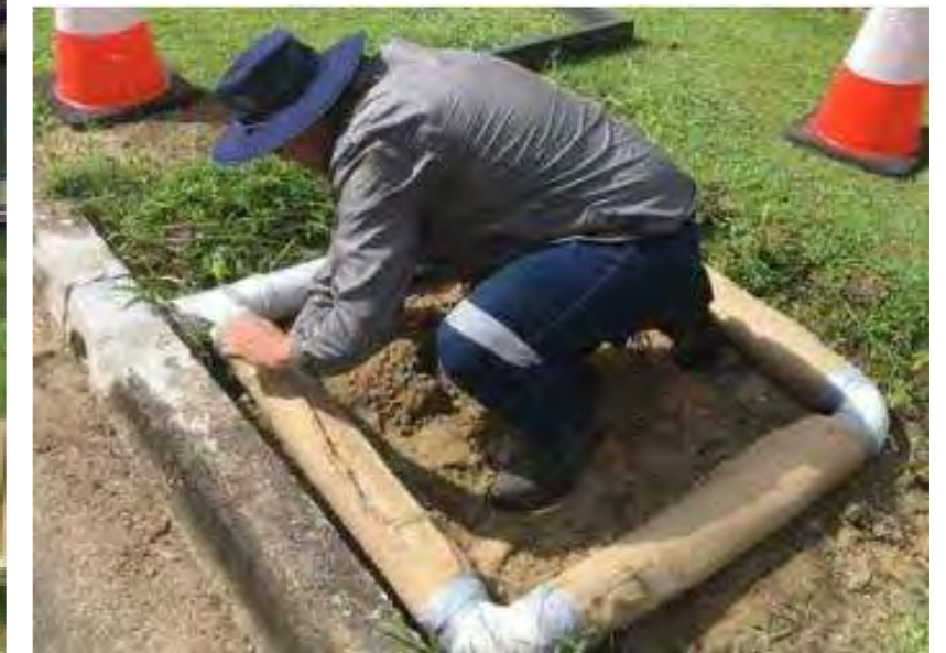
Images of example trees with leaky pipes – Source: Water By Design - Waterwise Street Tree Booklet
