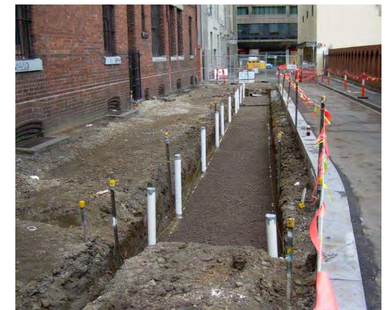
Godfrey St Infiltration trench under construction Source: http://urbanwater.melbourne.vic.gov.au/projects/greening-projects/godfrey-street-greening-project/
