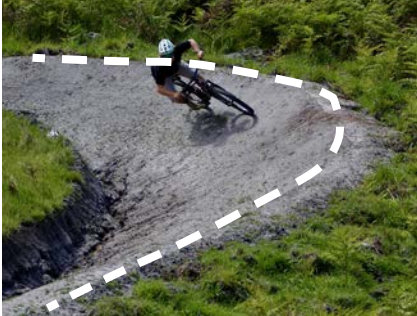
Berm corner. A bermed corner has a banked outer edge that runs the entire length of the corner to support the rider as they turn.
