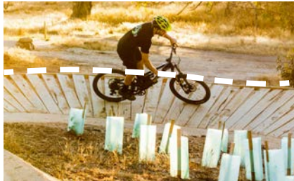
Berm. A berm is a banked corner in the track. They have an outer edge that runs the entire length of the corner to support the rider as they turn.
