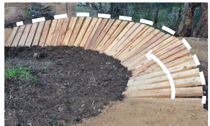
Wall ride. A curved extension to a berm that allows riders to ride up on the wall and jump off the end or flow back onto the track.
