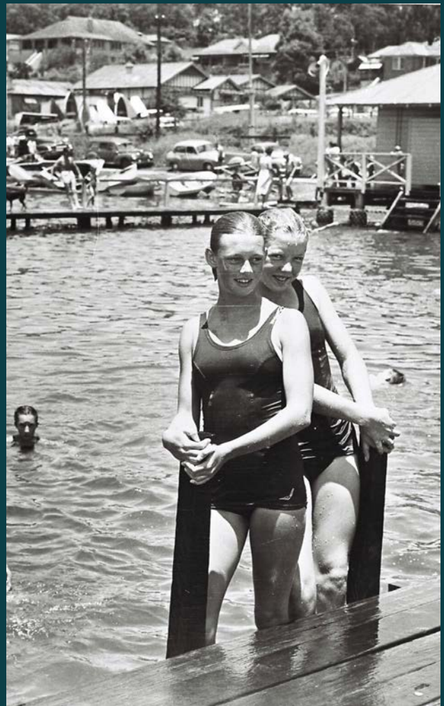
Toronto Baths under construction, Lake Macquarie, NSW (Lake Macquarie City Council)
