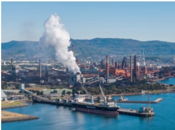
Figure 14. Portside factories in Port Kembla
