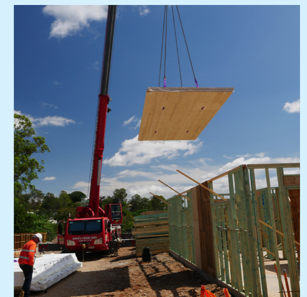
Accelerated construction Delivery of CLT floor slabs to site
