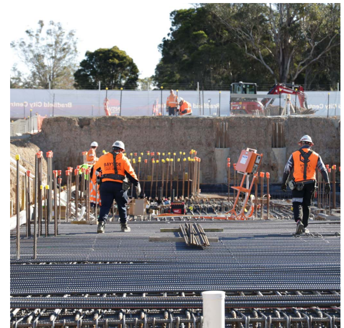
A building construction site, Badgery's Creek Road, Bringelly
